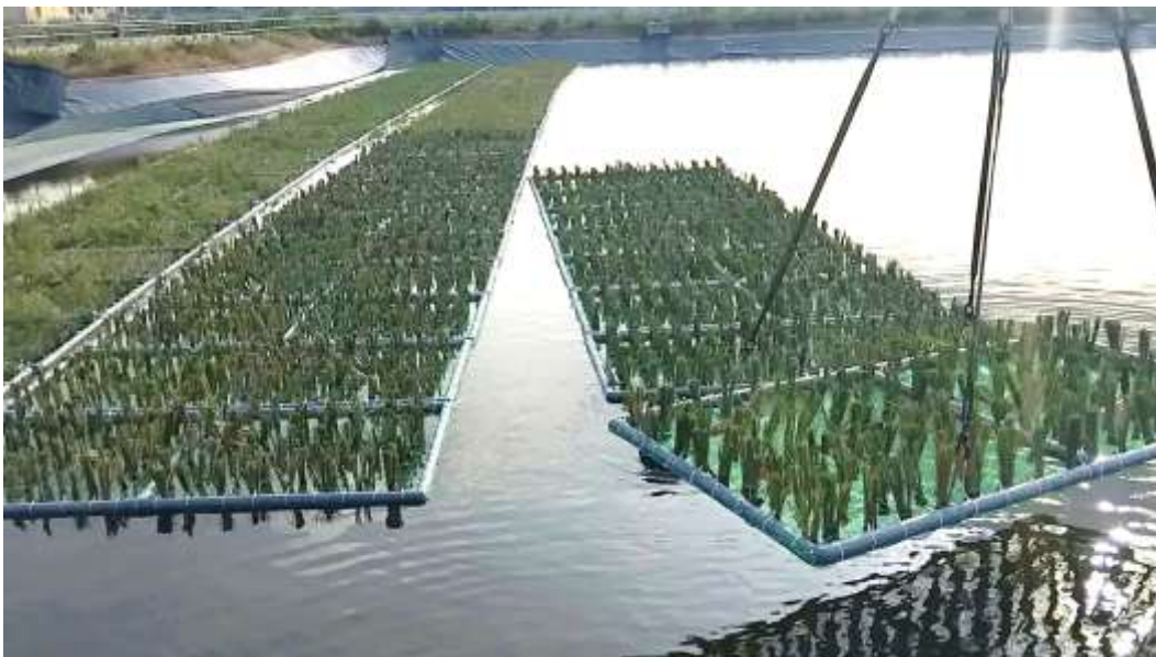
Photo 5: A planted raft being lowered by sling into the lagoon and joined to the end of a strip of rafts already afloat. Photo: OlaFarm (olafarm.com), used with permission.
