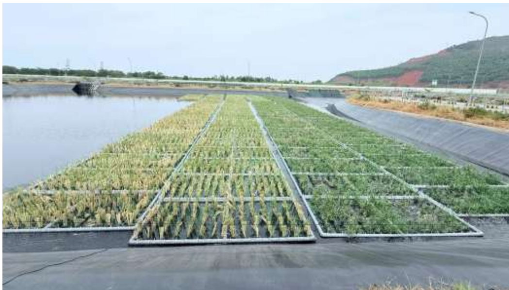
Photo 1: Strips of floating rafts planted with vetiver and umbrella sedge on the refinery's lined lagoon. Newly planted vetiver rafts, still yellow, lie next to rafts that have already greened. The project used both species: 60% vetiver, 40% umbrella sedge. Photo: OlaFarm (olafarm.com), used with permission.
