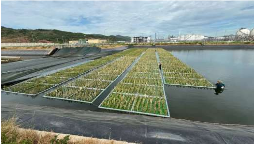
Photo 8: Workers wading in the lagoon to tow and tie newly launched vetiver and sedge rafts into neat strips, with the refinery and storage tanks in the distance. Photo: OlaFarm (olafarm.com), used with permission.
