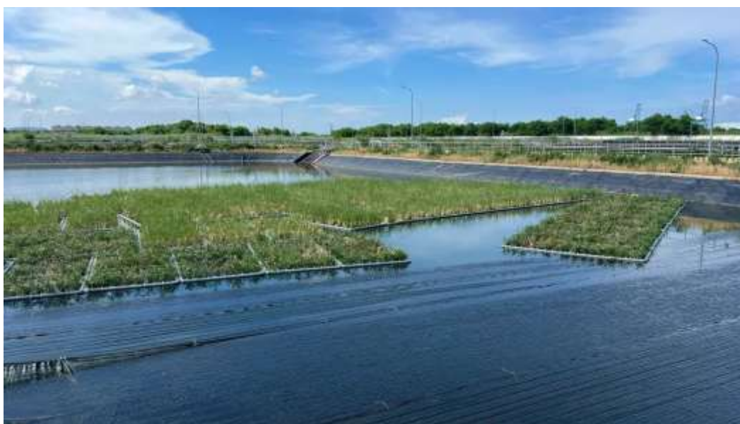
Photo 2: Vetiver and umbrella sedge rafts side by side on the black-lined lagoon, with railings and pipelines along the bank and port cranes on the horizon. Rafts about six weeks after planting. Photo: OlaFarm (olafarm.com), used with permission.
