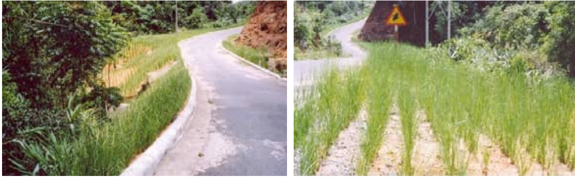
Slope stabilization at Ba Na road
