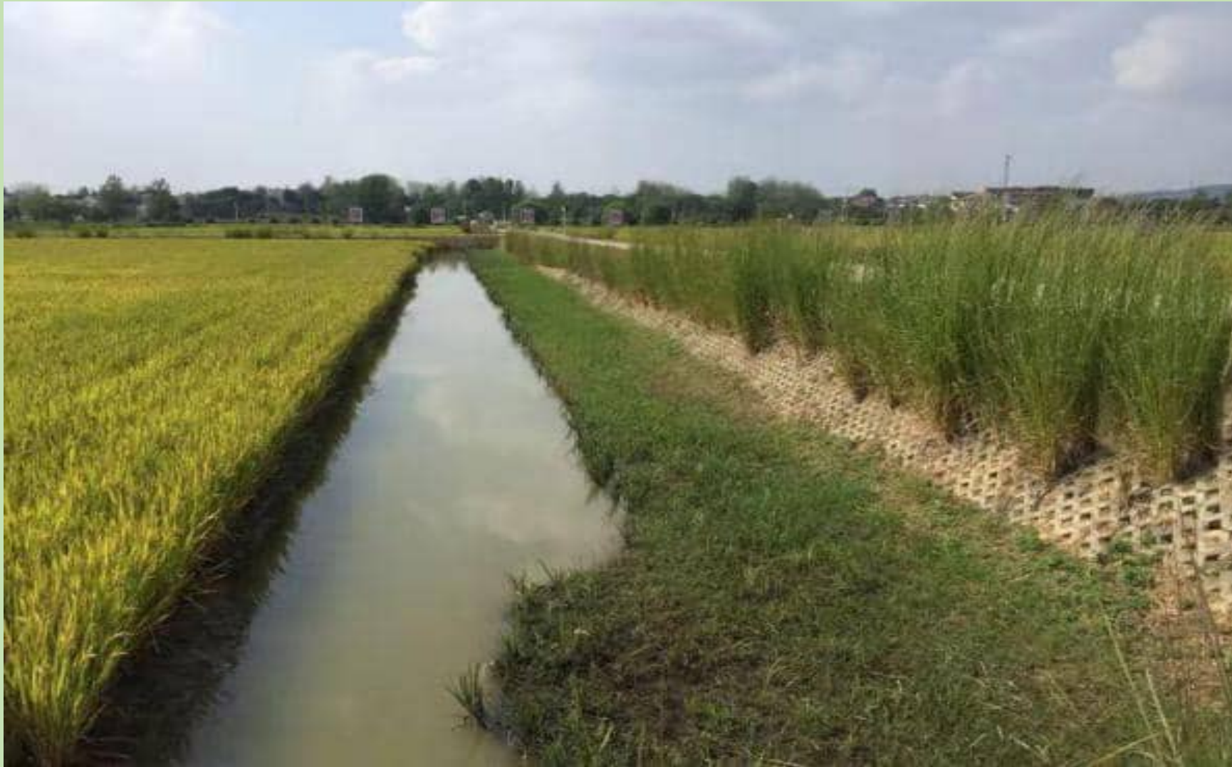
Vetiver for cement blocks fixing
