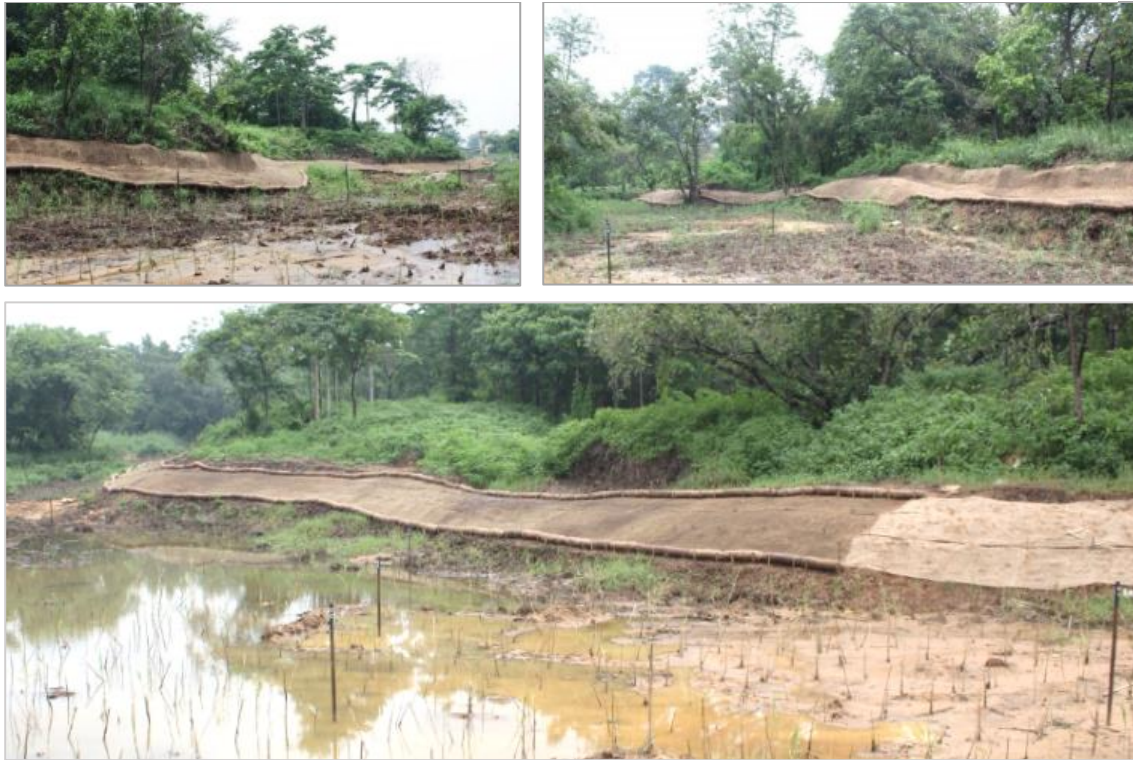
Phase – 2 – Slope preparation & Jute Geotextiles application
