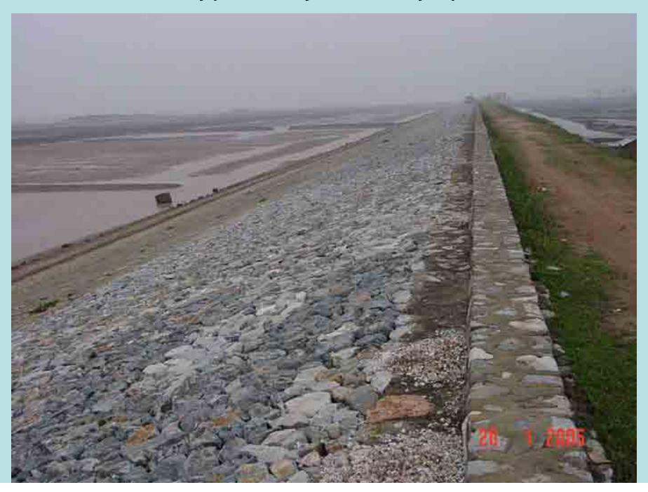
But this new dike, although its outside batter protected by the extremely expensive rock armour;, its inside batter was not protected, cover only by local vegetation, mostly weeds
