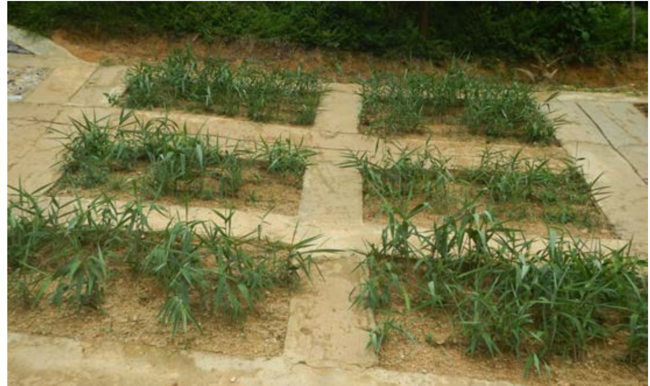
Masonry framework with grass on cut slope at SP35 in Thai Nguyen Province one month after plantation
