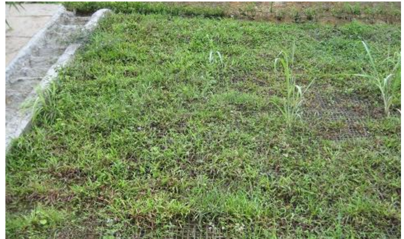
Bamboo mesh and short grass ten months after plantation on cut slope at SP35 in Thai Nguyen Province
