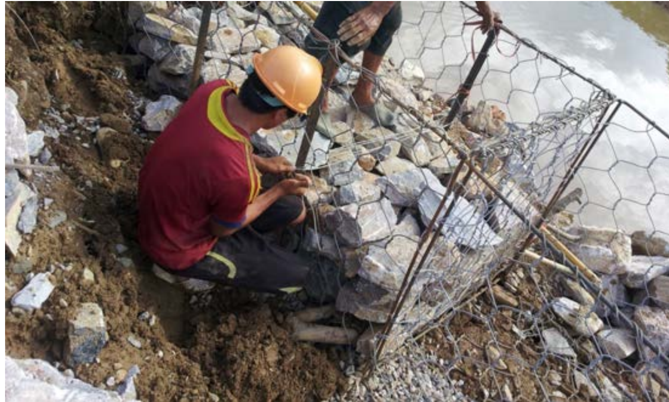
Constructing vegetated gabions in riverbank embankment at SP32 in Son La Province
