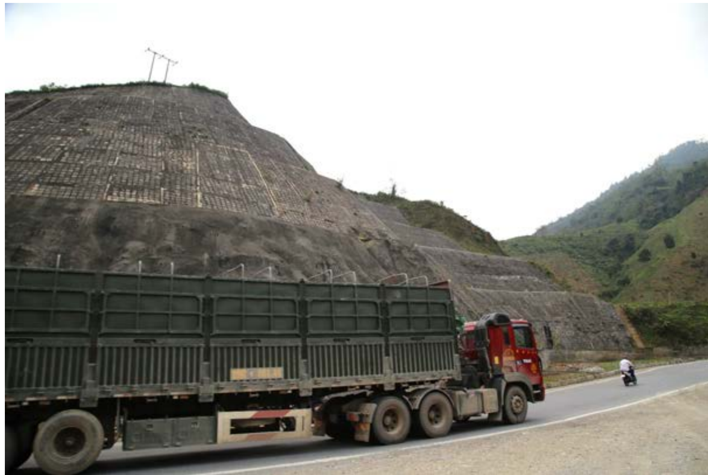
Hard techniques protecting slope in national highway from Hoa Binh Province to Son La Province
