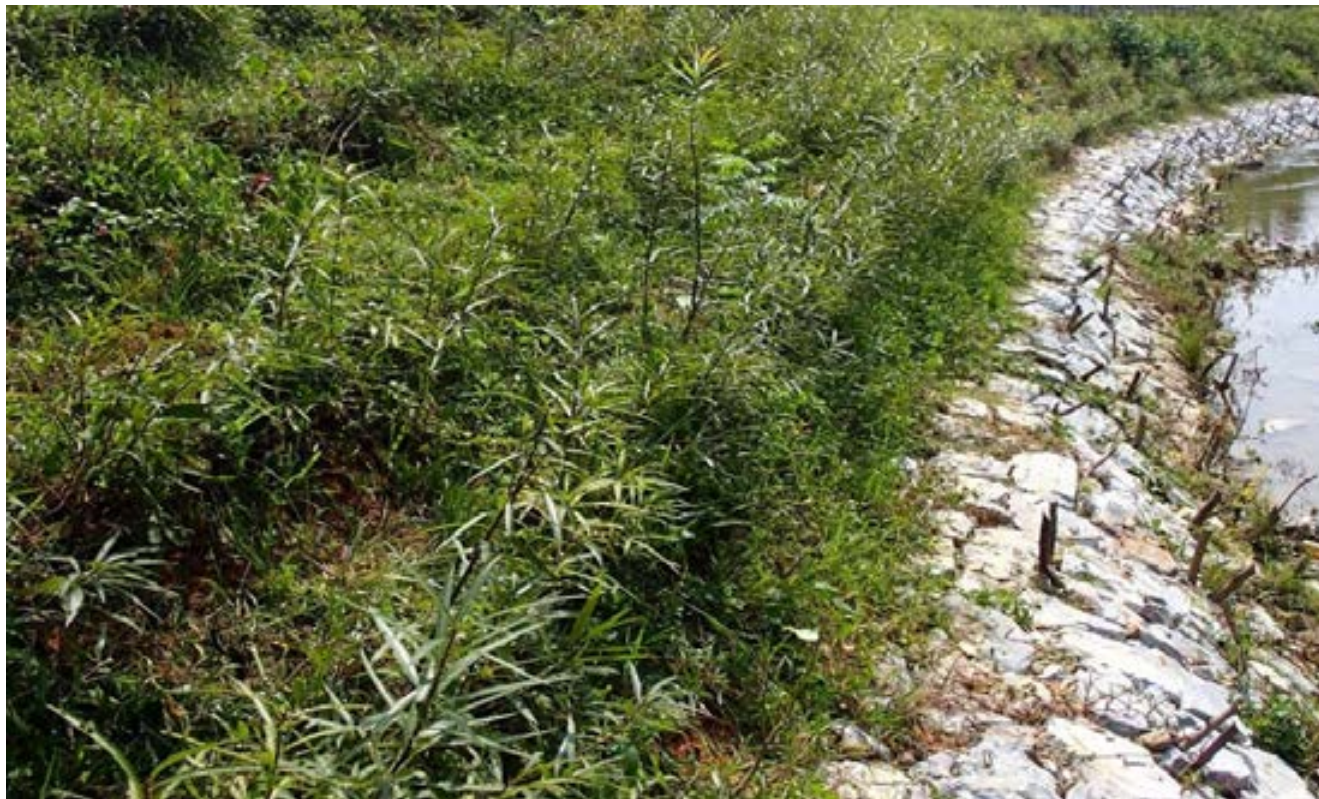
Brush layers in riverbank embankment at SP4 in Bac Kan Province four months after plantation
