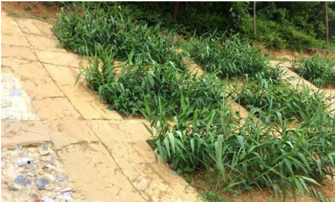
Masonry framework with grass on cut slope at SP35 in Thai Nguyen Province two months after plantation
