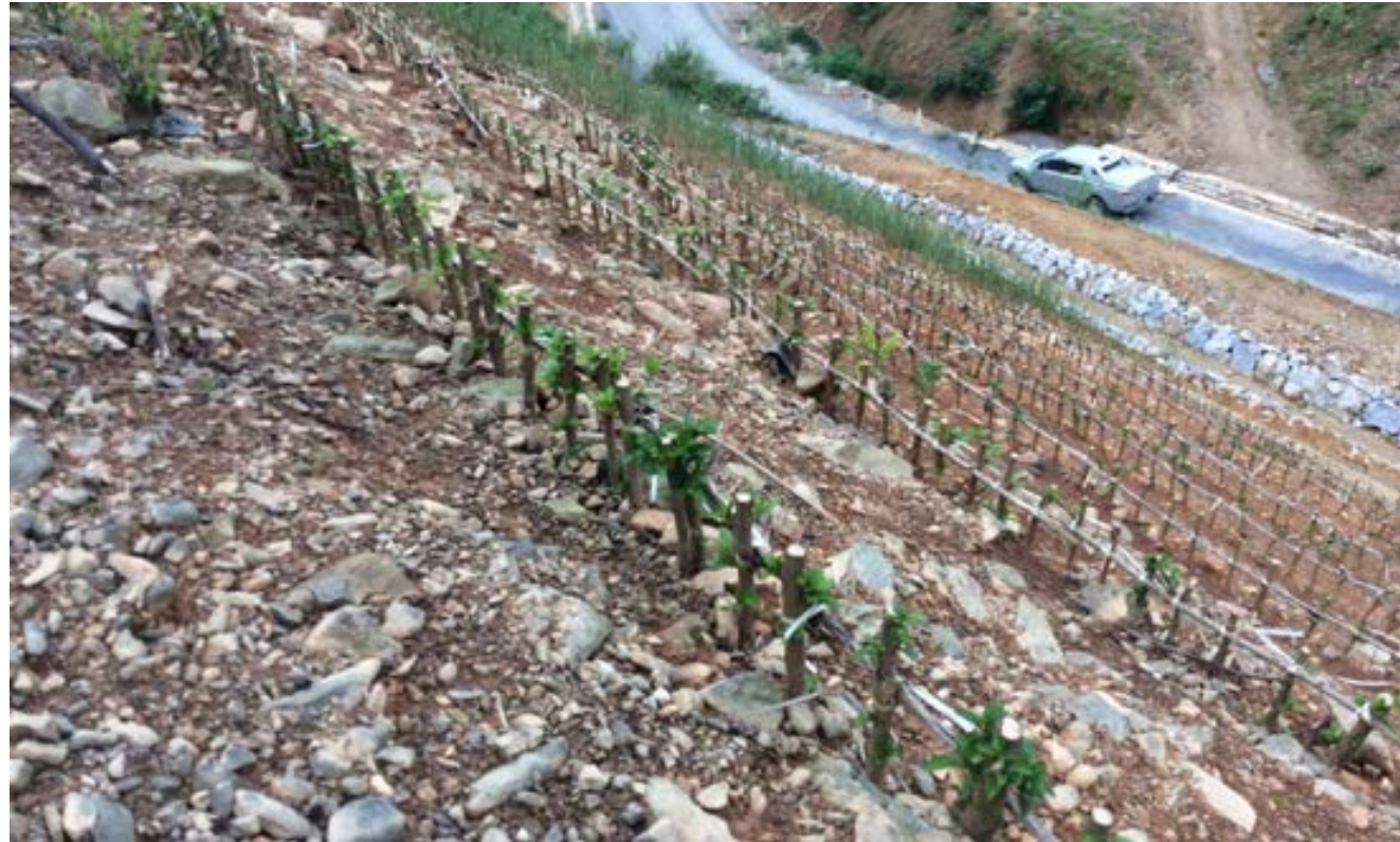
Newly planted palisades on cut slope at SP35 in Thai Nguyen Province
