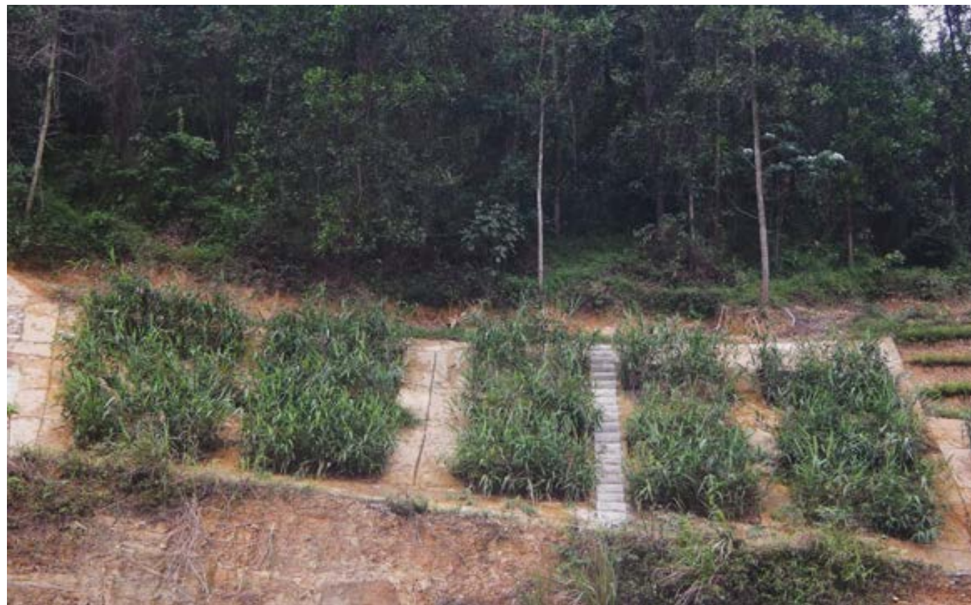
Masonry framework with grass on cut slope at SP35 in Thai Nguyen Province
