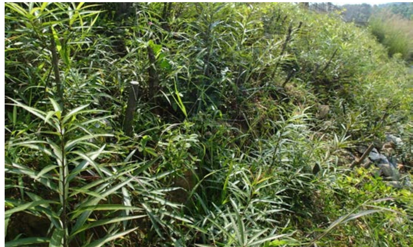
Willow-leaved water croton used to construct live poles in riverbank embankment at SP4 in Bac Kan Province
