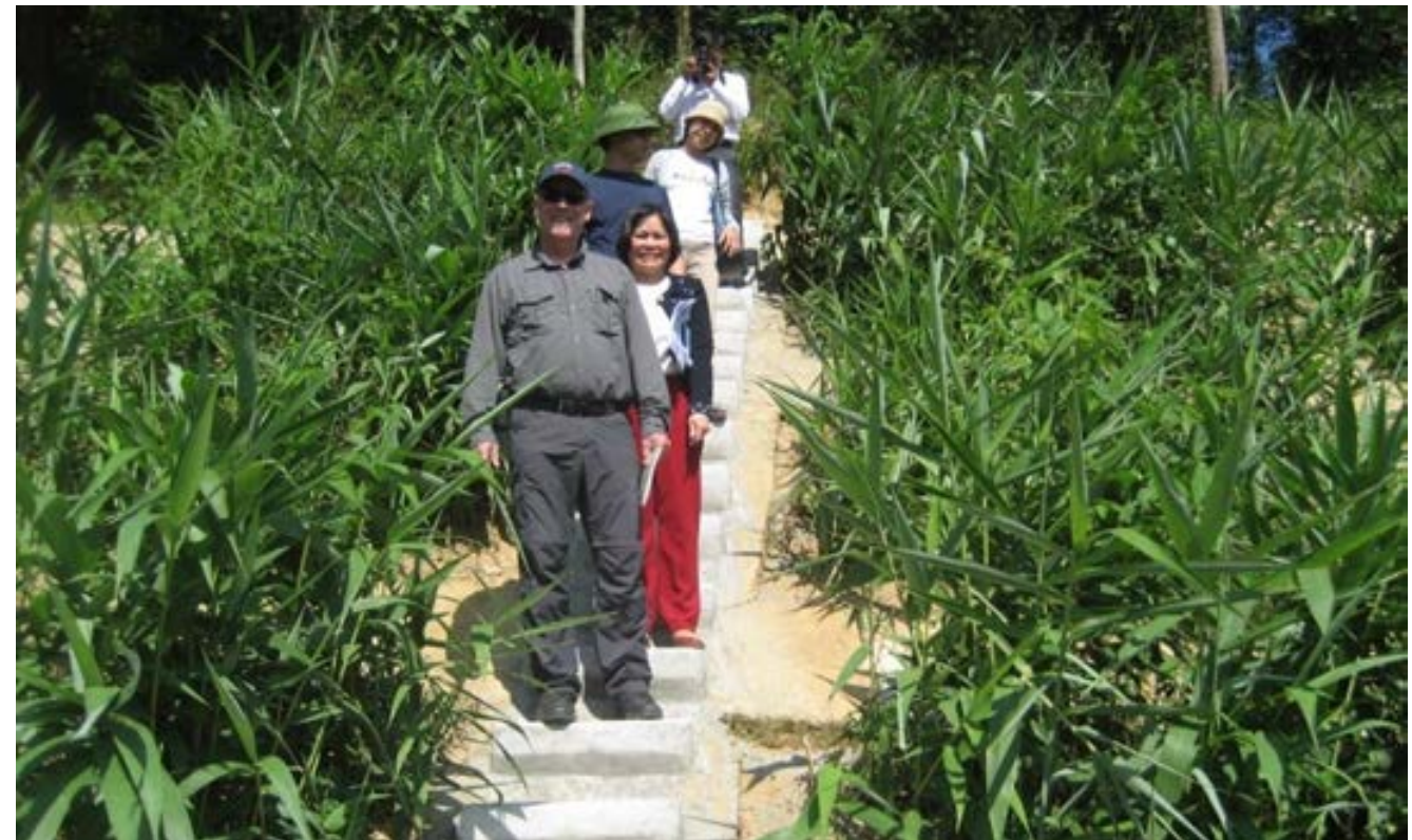
Masonry framework with grass on cut slope at SP35 in Thai Nguyen Province five months after plantation
