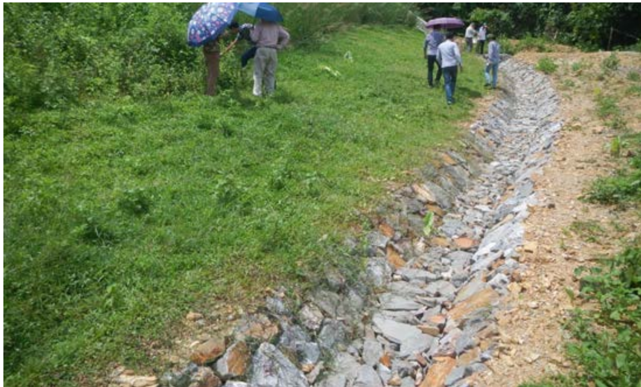
Dry stone pitching to drainage channel at the toe of fill slope at SP35 in Thai Nguyen Province
