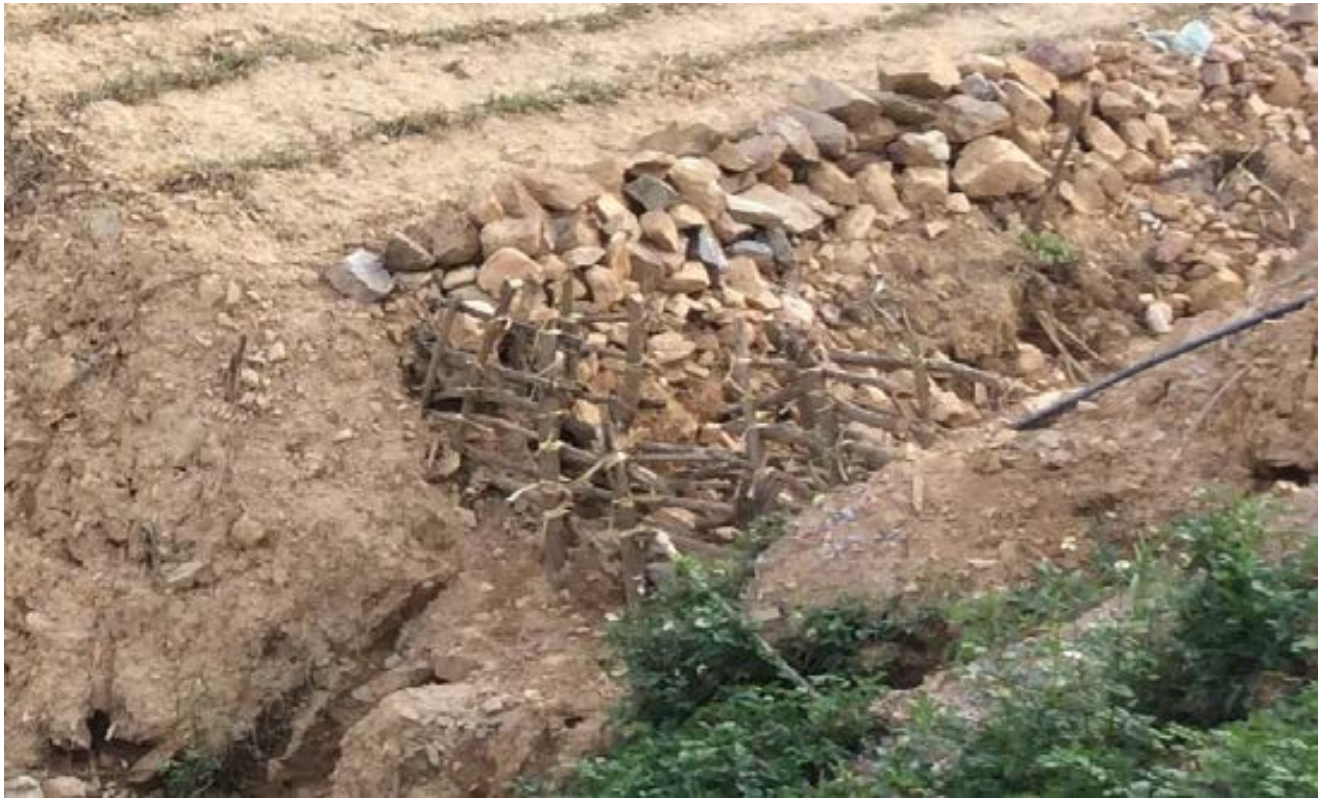
Newly constructed live check dam at the base of fill slope at SP35 in Thai Nguyen Province
