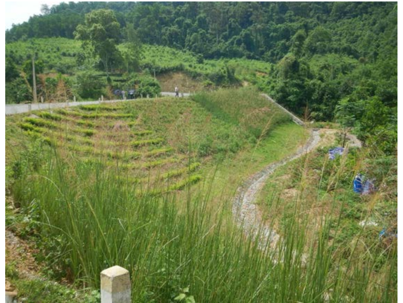
Vegetative techniques protecting fill slope at SP35 in Thai Nguyen Province
