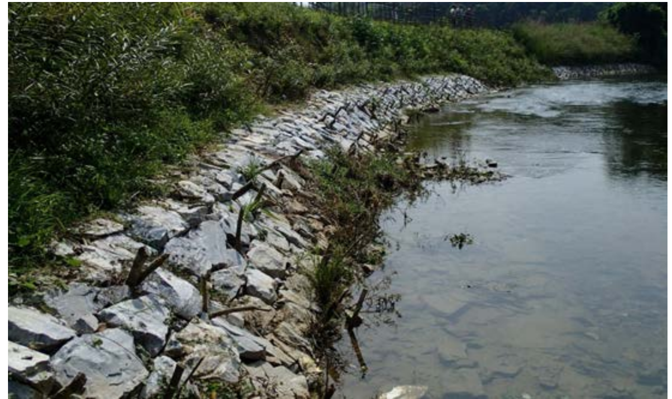
Vegetated riprap protecting the toe of riverbank at SP4 in Bac Kan Province
