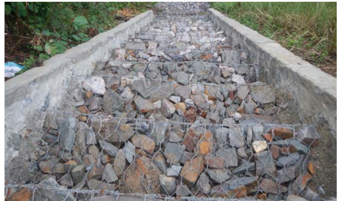
Gabion cascade on fill slope at SP35 in Thai Nguyen Province
