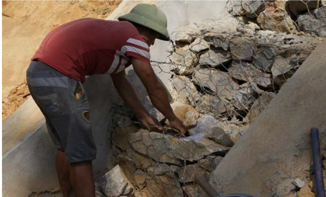
Constructing gabion cascade on cut slope at SP31 in Son La Province
