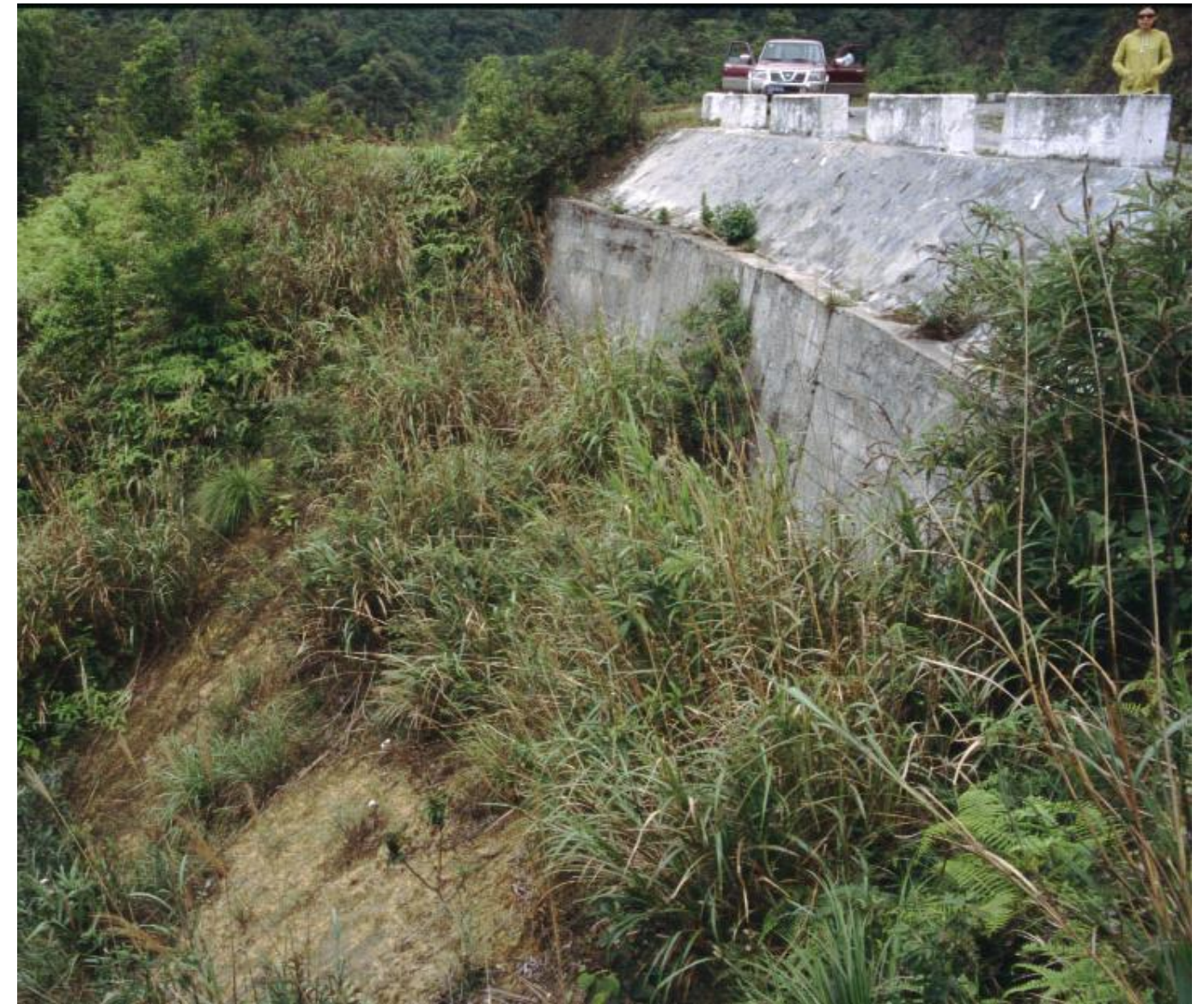
Figure 6. A rehabilitated valley side slope on a mountain road in Sa Pa. The project's demonstration trials show that one worker can plant 4 m 2 of large grasses per day.
