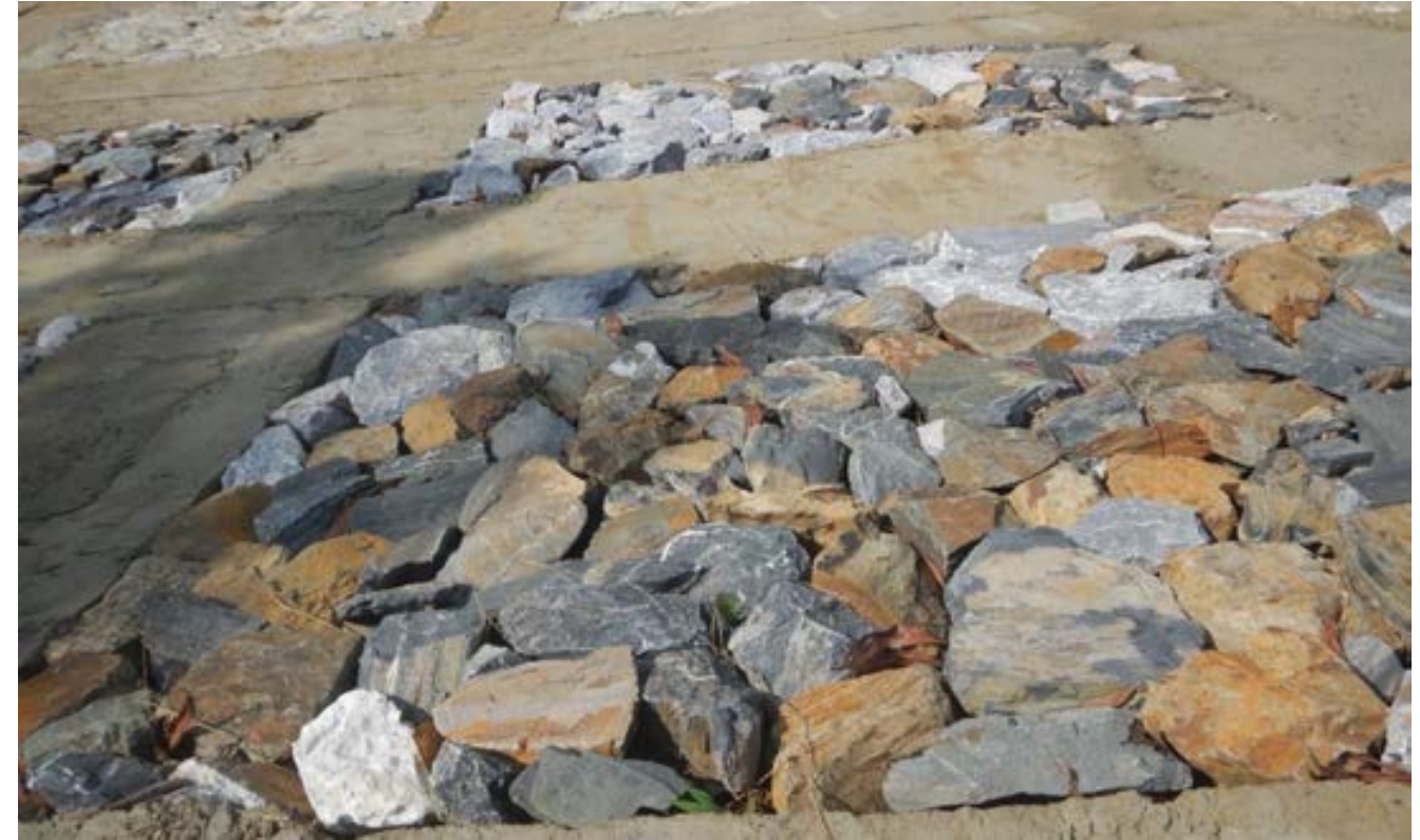
Dry stone infill used on cut slope at SP35 in Thai Nguyen Province
