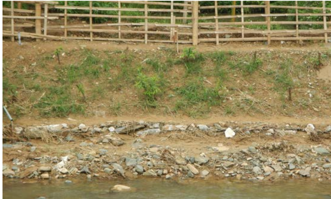
Newly planted live poles in riverbank embankment at SP32 in Son La Province
