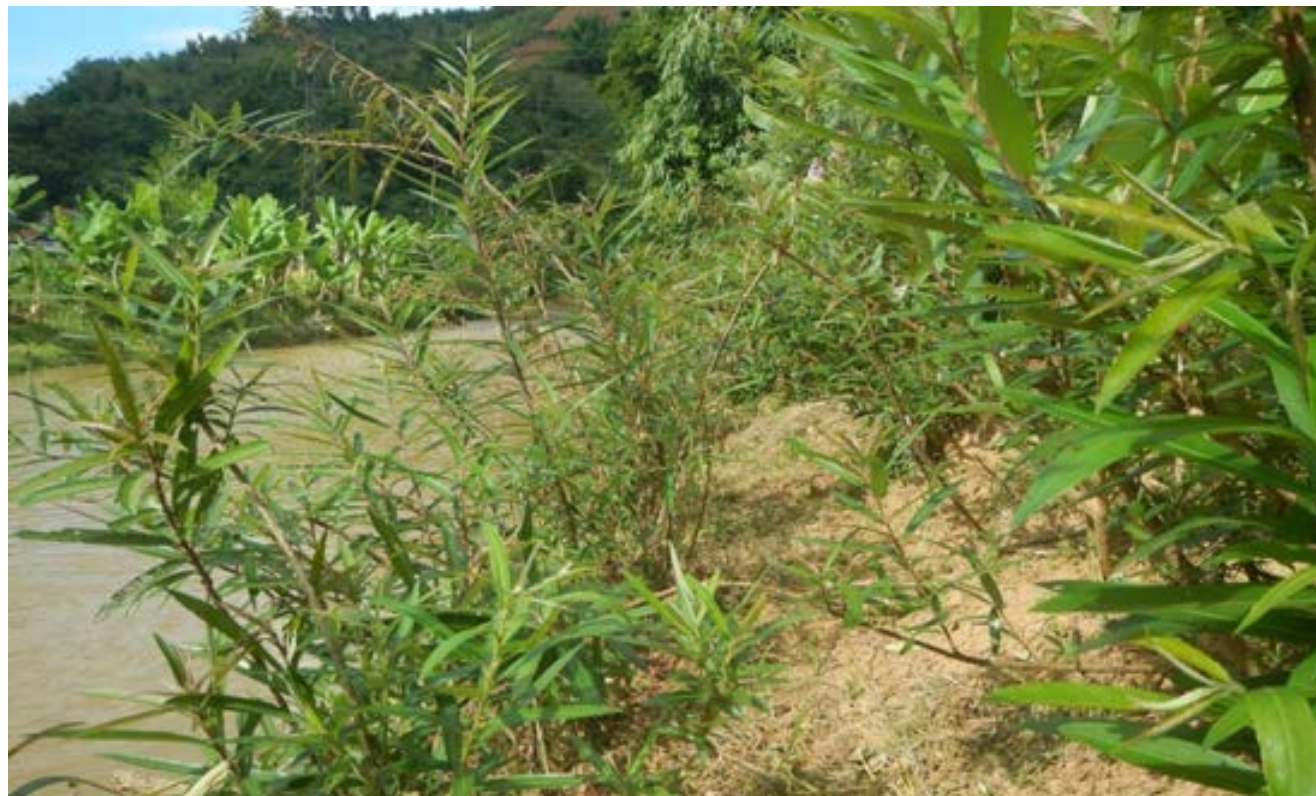
Live fences in riverbank embankment at SP32 in Son La Province after 14 months and three flood seasons
