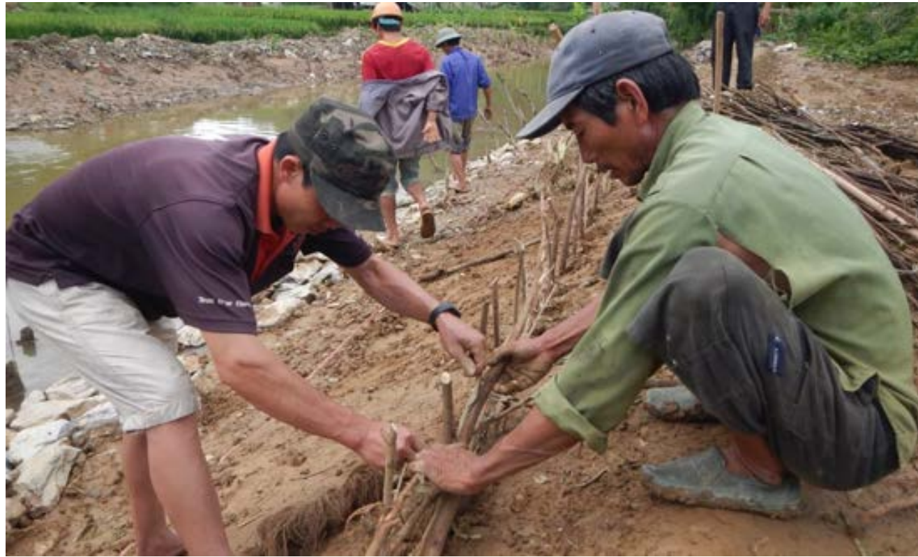
Constructing live fences in riverbank embankment at SP32 in Son La Province
