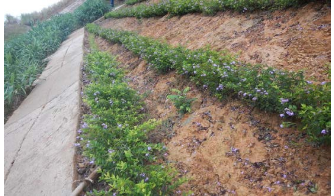
Brush layers on cut slope at SP35 in Thai Nguyen Province two months after plantation
