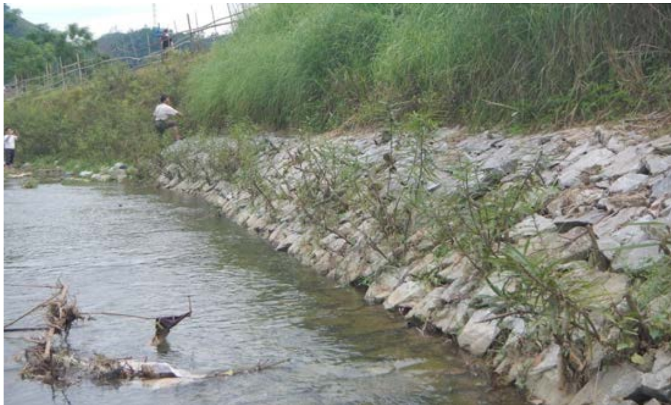
Vegetated riprap protecting the toe of riverbank at SP4 in Bac Kan Province 13 months after plantation
