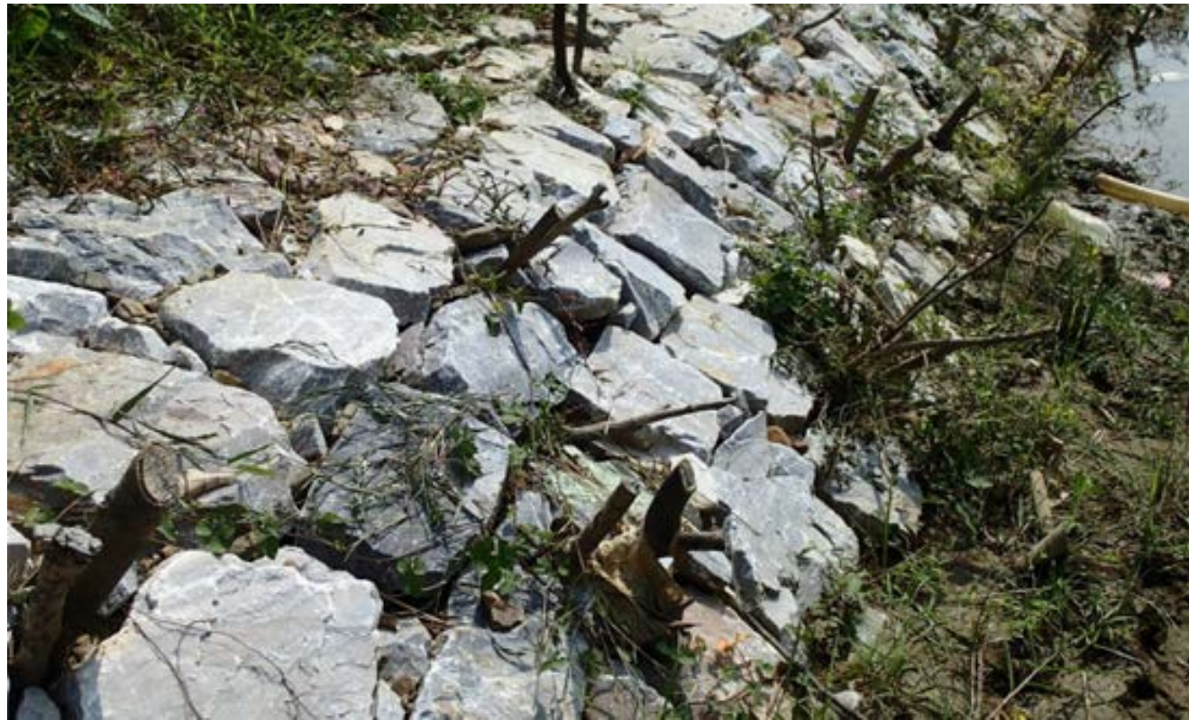
Vegetated riprap in riverbank embankment at SP4 in Bac Kan Province four months after plantation
