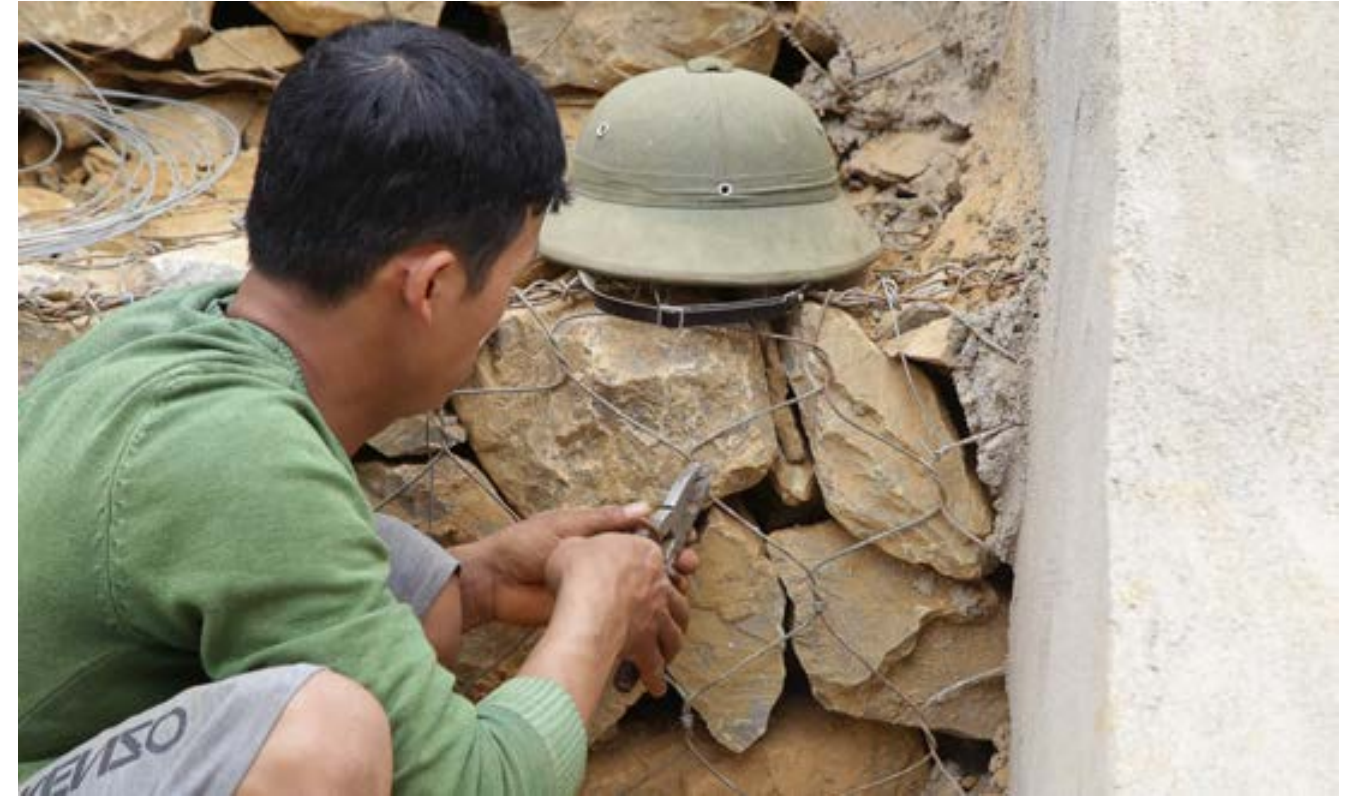
Constructing gabion cascade on cut slope at SP31 in Son La Province
