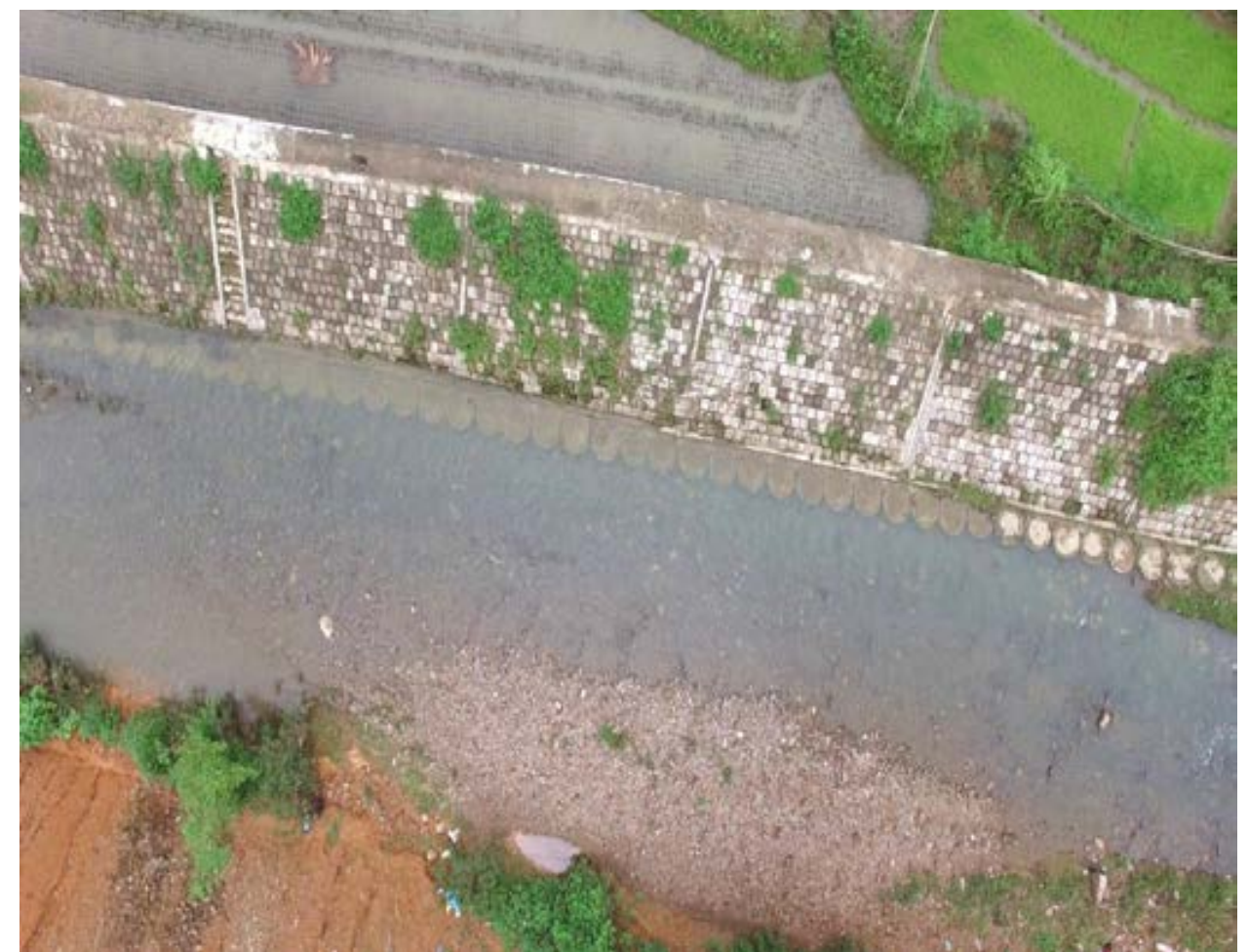
Conventional revetment protecting riverbank at SP4 in Bac Kan Province
