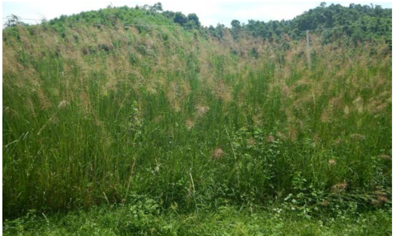
Vetiver grass lines on fill slope embankment at SP35 in Thai Nguyen Province three months after plantation
