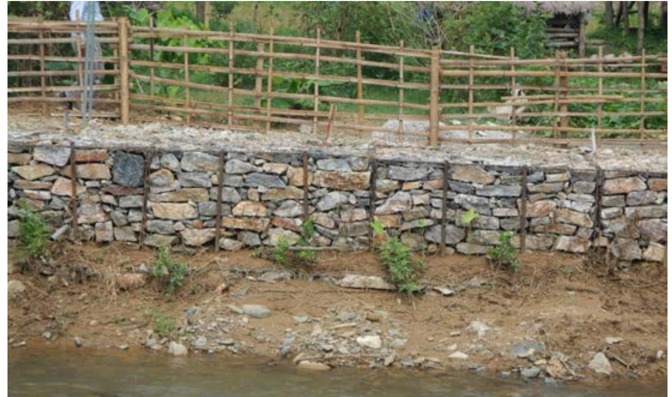
Completed vegetated gabions in riverbank embankment at SP32 in Son La Province
