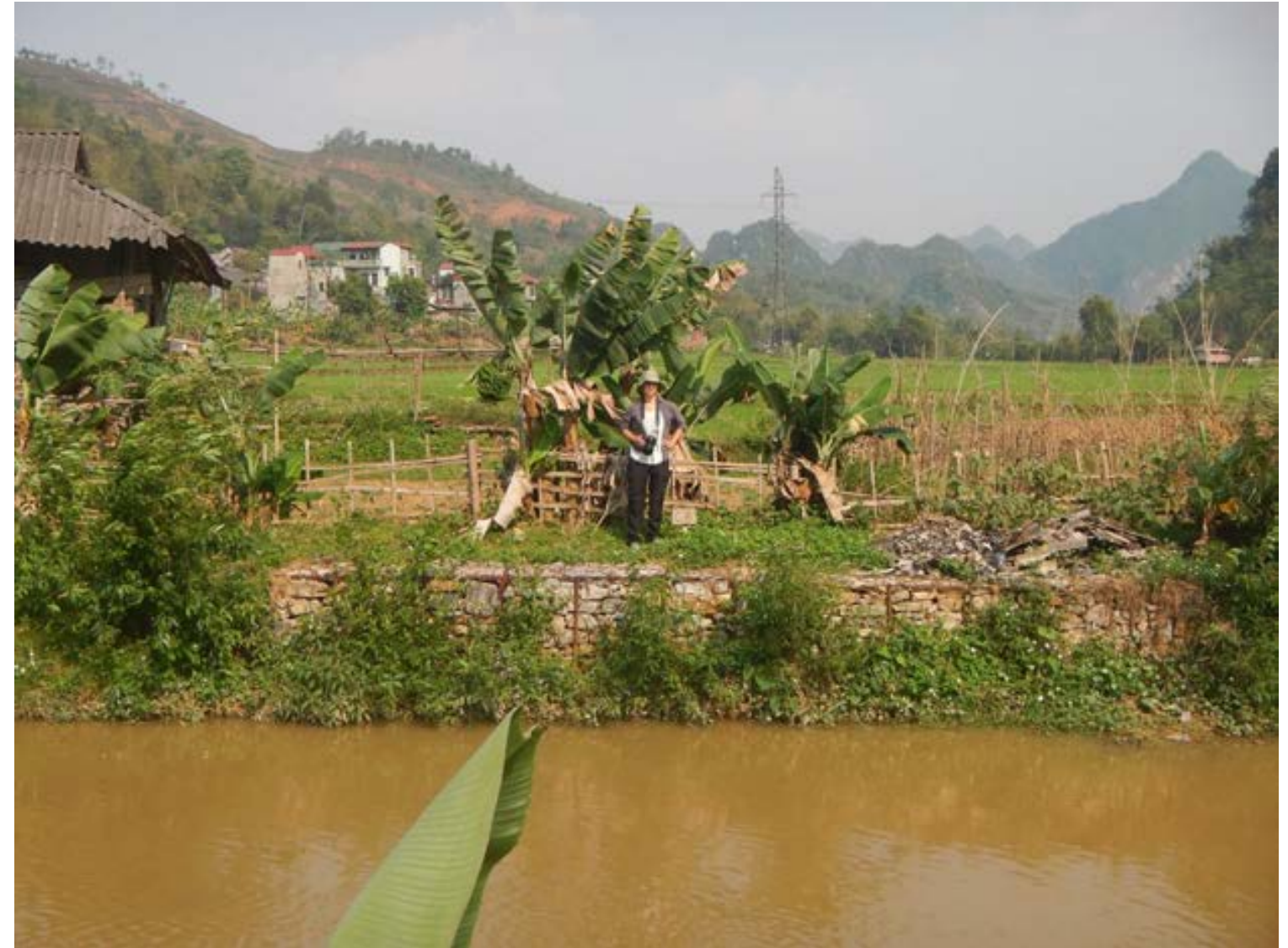
Plants growing through layers of rock in vegetated gabion technique at riverbank embankment at SP32 in Son La Province, providing flexible binding to the structure once the wire has corroded
