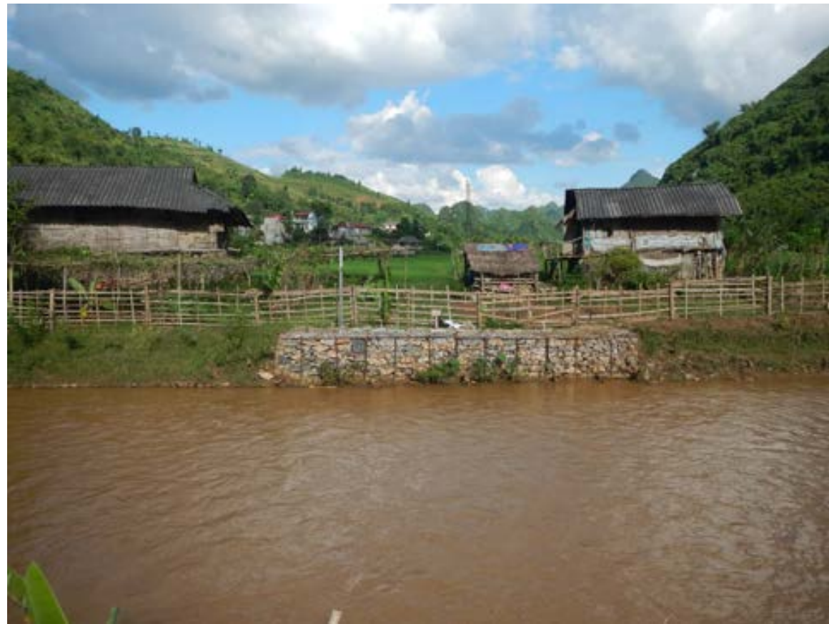
Vegetated gabion technique protecting riverbank together with live poles and live fences techniques at SP32 in Son La Province
