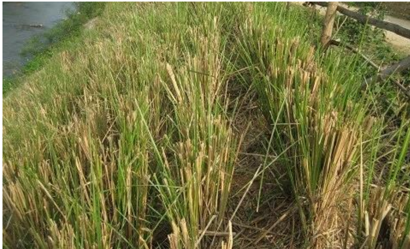
Operation and maintenance of Vetiver grass in riverbank embankment at SP4 in Bac Kan Province
