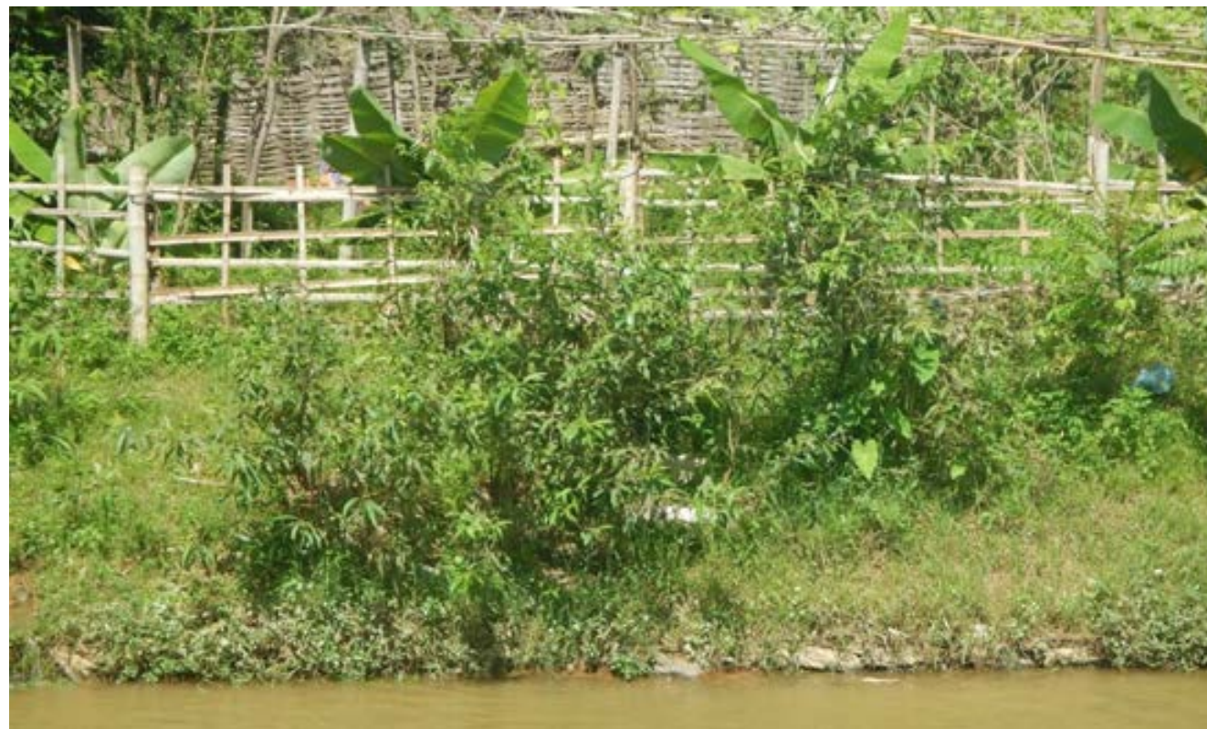
Live poles in riverbank embankment at SP32 in Son La Province after one year and two flood seasons
