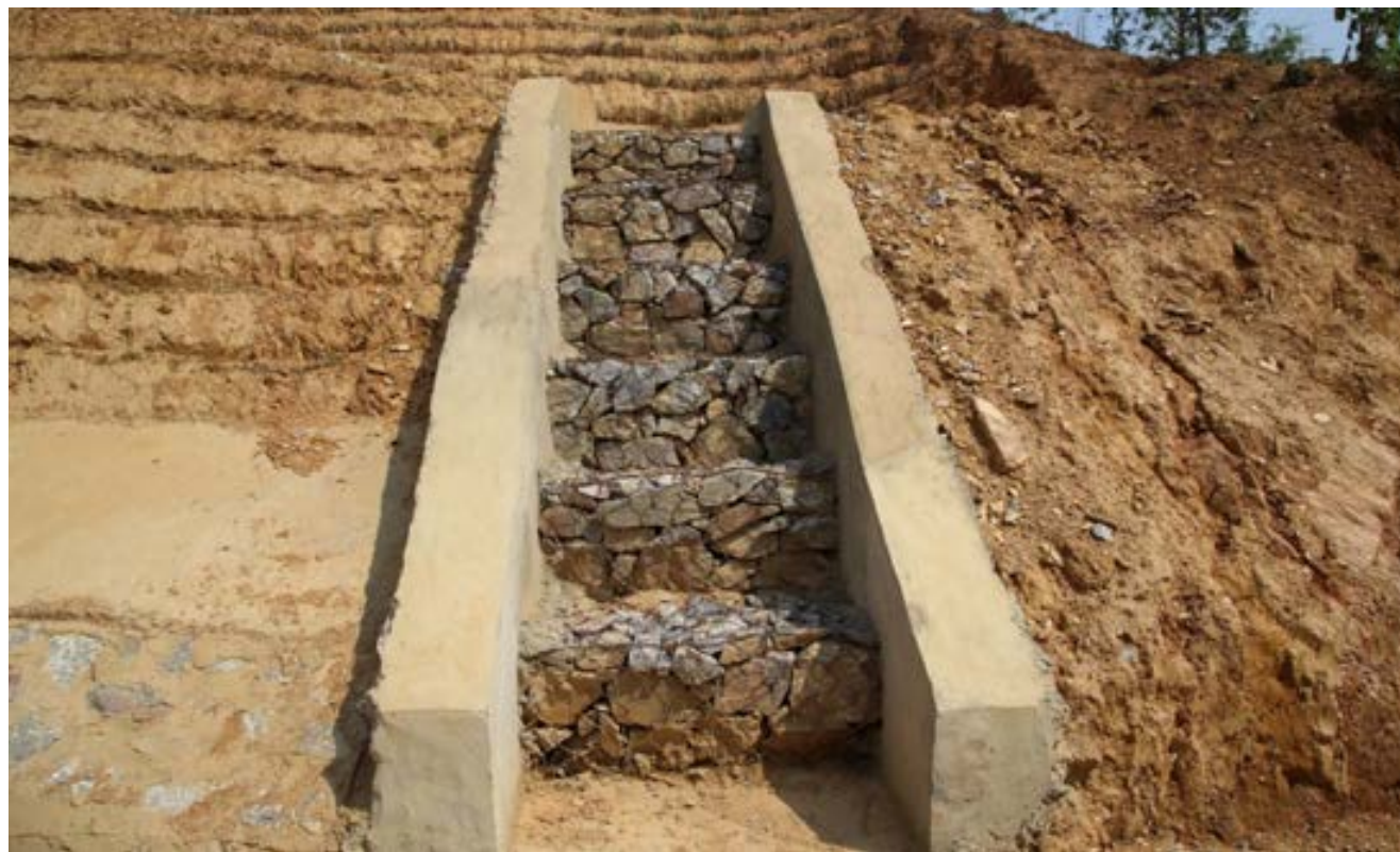
Gabion cascade on cut slope at SP31 in Son La Province
