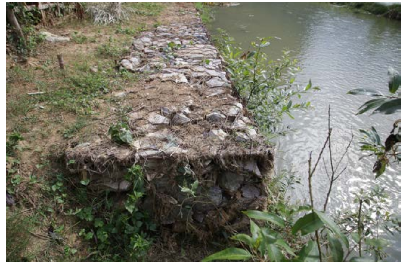
Vegetated gabions protecting riverbank at SP32 in Son La Province
