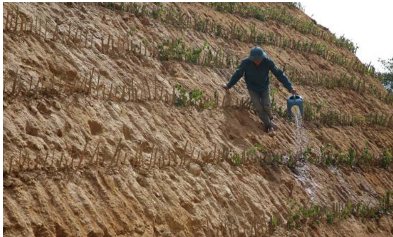
Watering palisades on cut slope at SP31 in Son La Province
