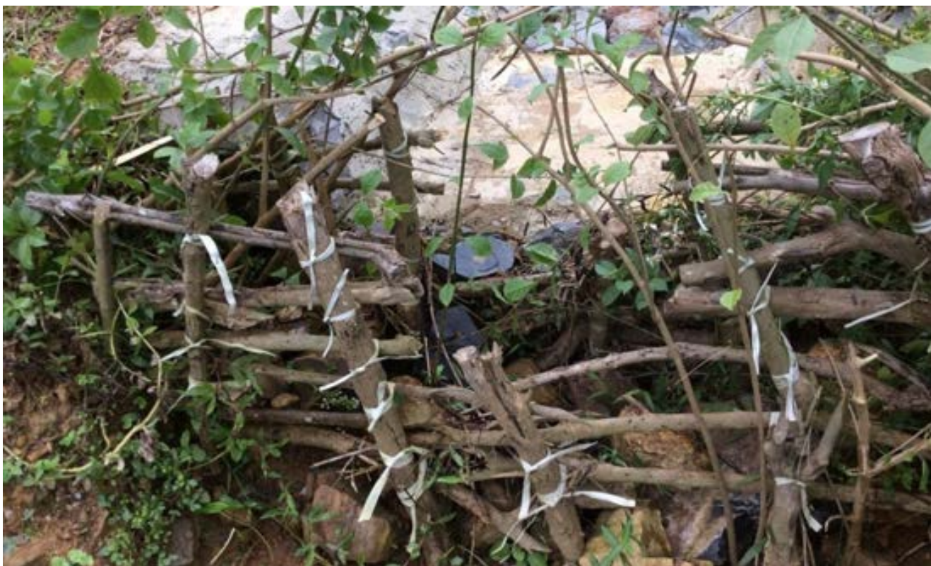
Live check dam on fill slope at SP35 in Thai Nguyen Province after replantation
