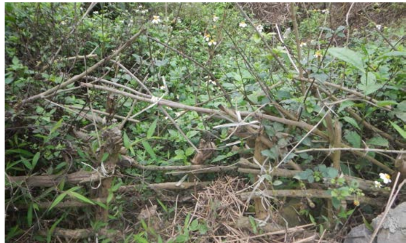
Live check dam on fill slope at SP35 in Thai Nguyen Province five months after replantation
