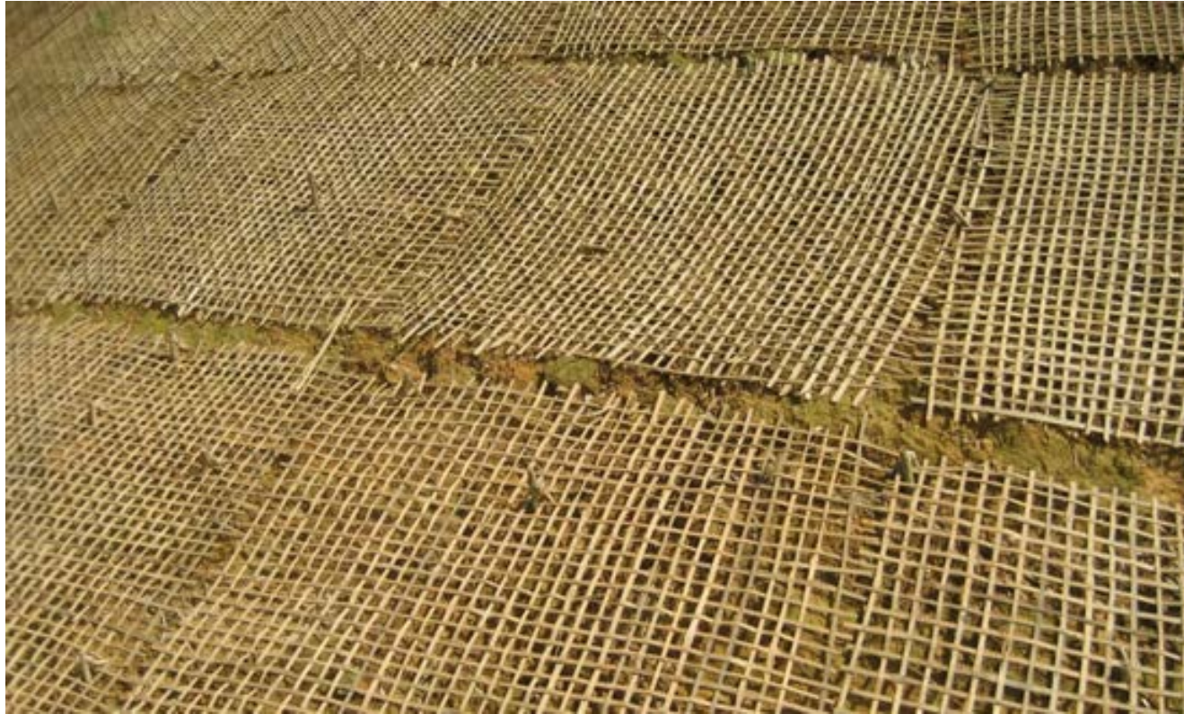
Bamboo mesh laid out on cut slope at SP35 in Thai Nguyen Province
