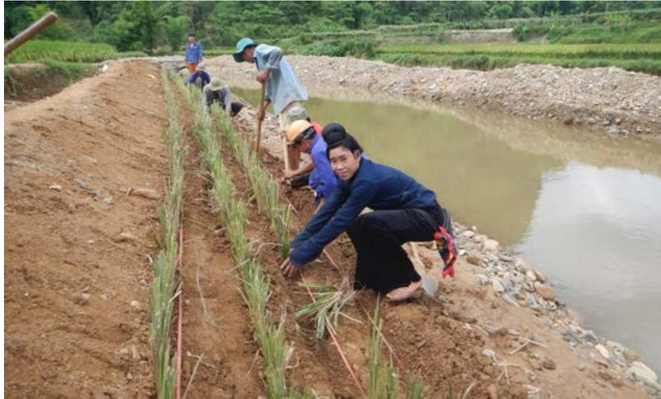
Planting Vetiver grass in riverbank embankment site at SP32 in Son La province
