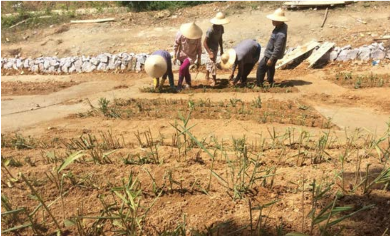
Constructing masonry framework with grass on cut slope at SP35 in Thai Nguyen Province
