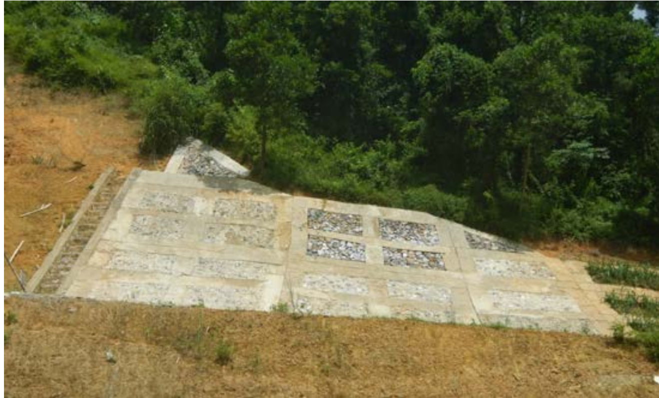
Masonry framework with dry stone infill on cut slope at SP35 in Thai Nguyen Province
