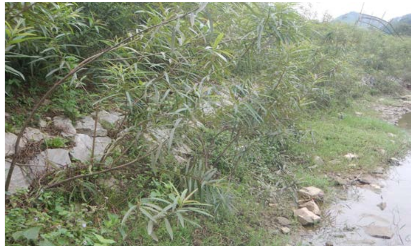
Vegetated riprap protecting the toe of riverbank at SP4 in Bac Kan Province 23 months after plantation
