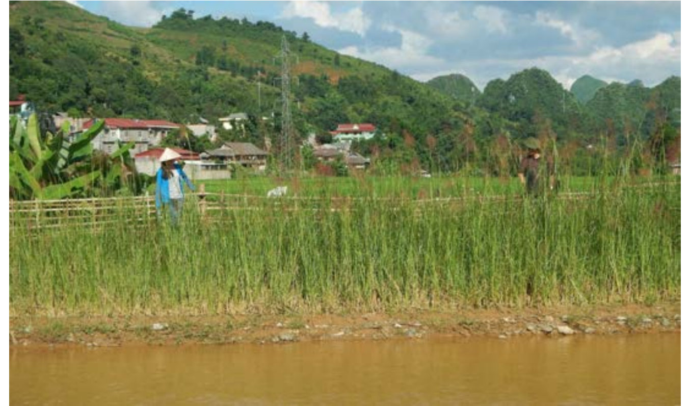
Vetiver grass lines in riverbank embankment at SP32 in Son La Province three months after plantation
