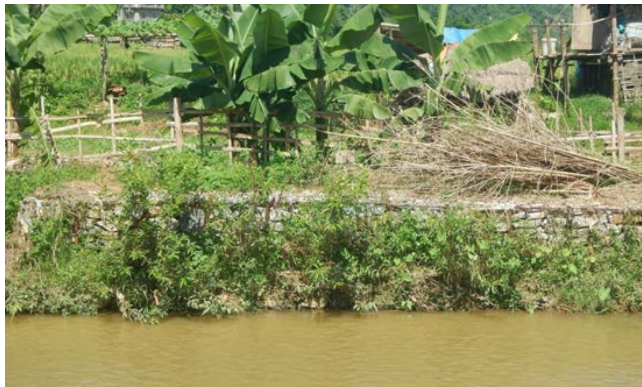
Vegetated gabions in riverbank embankment at SP32 in Son La Province after one year and two flood seasons
