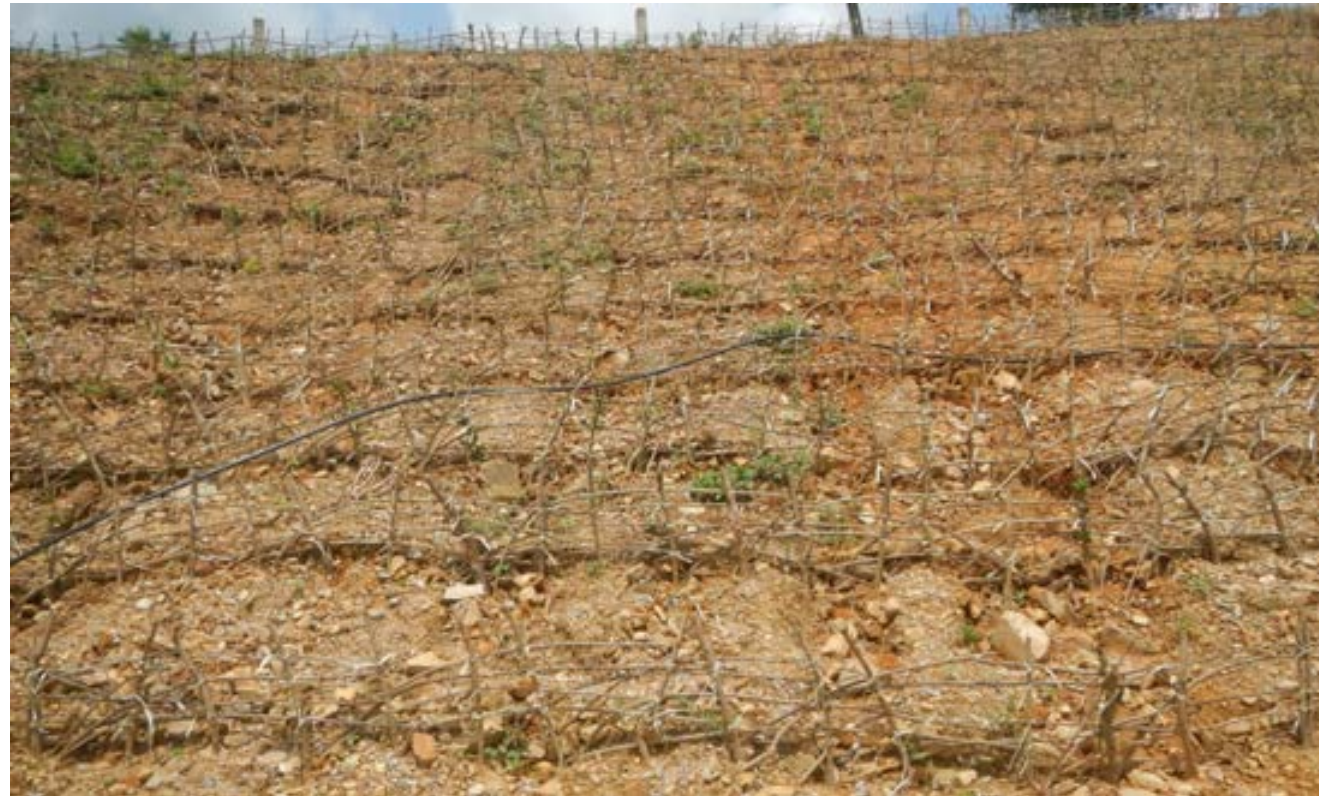
Fascines in early development on fill slope at SP35 in Thai Nguyen Province
