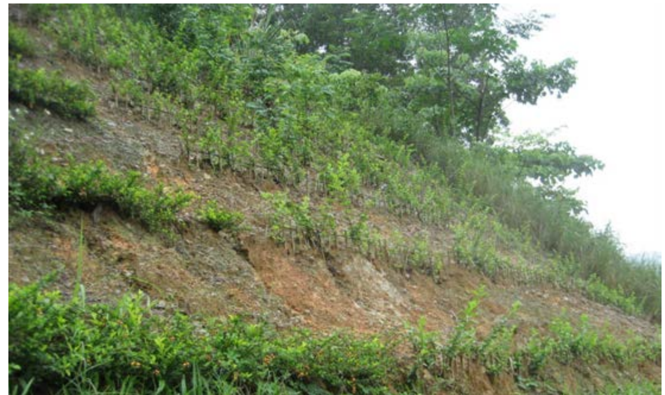
Palisades on cut slope at SP35 in Thai Nguyen Province ten months after plantation
