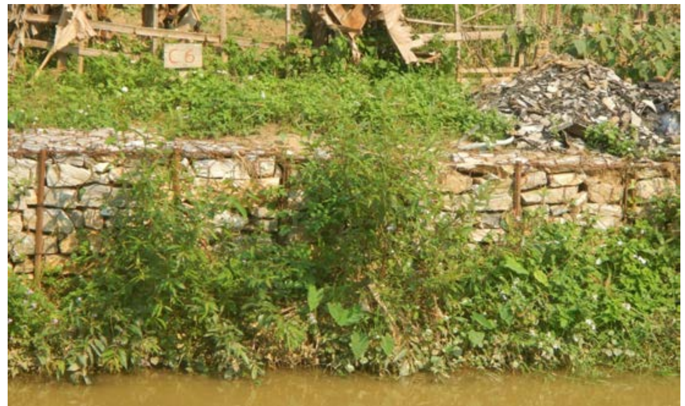
Vegetated gabions in riverbank embankment at SP32 in Son La Province after 21 months and three flood seasons
