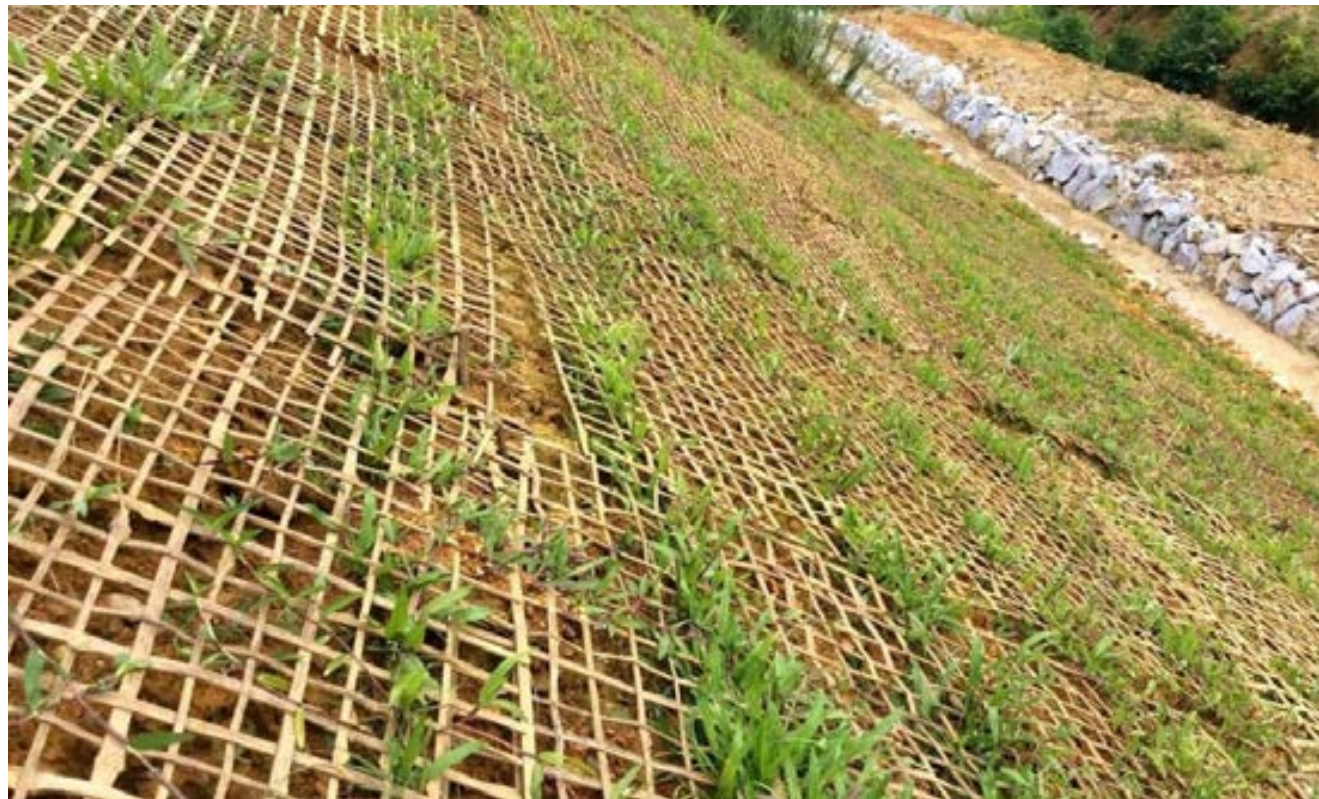
Bamboo mesh and short grass one month after plantation on cut slope at SP35 in Thai Nguyen Province
