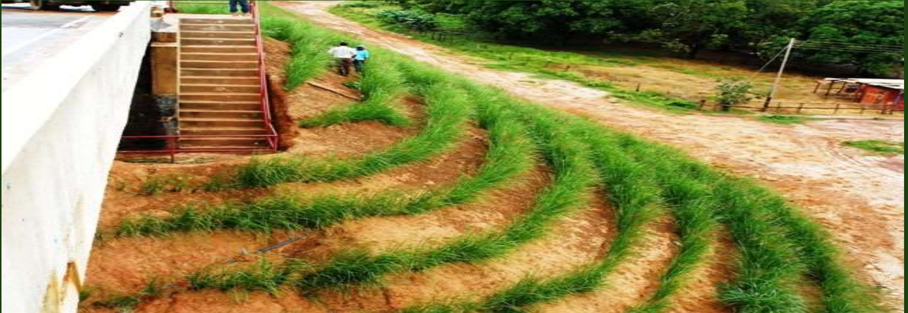
HIGHWAY BATTER STABILISATION
