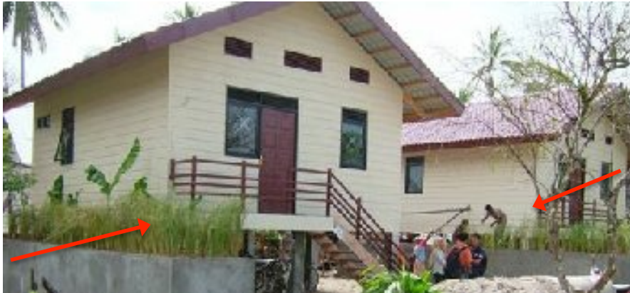
Banda Aceh Rehab – Indonesia - Domestic septic tank tertiary treatment
