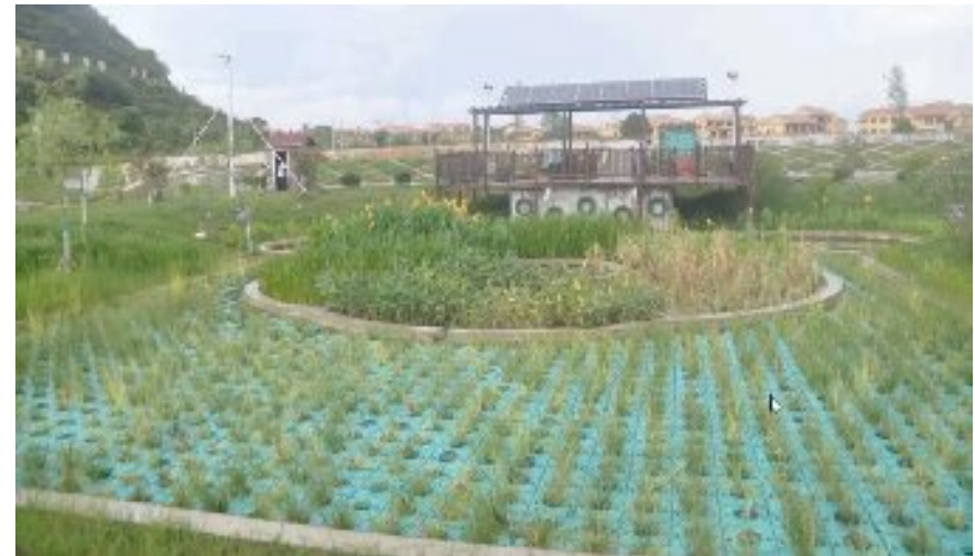
Floating treatment of tertiary sewage effluent - China
