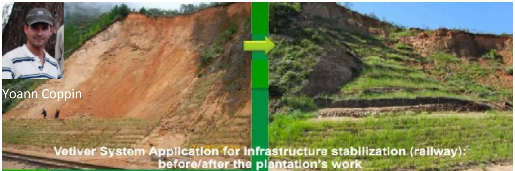
Madagascar - Extreme erosion and landslides Before and after vetiver application
