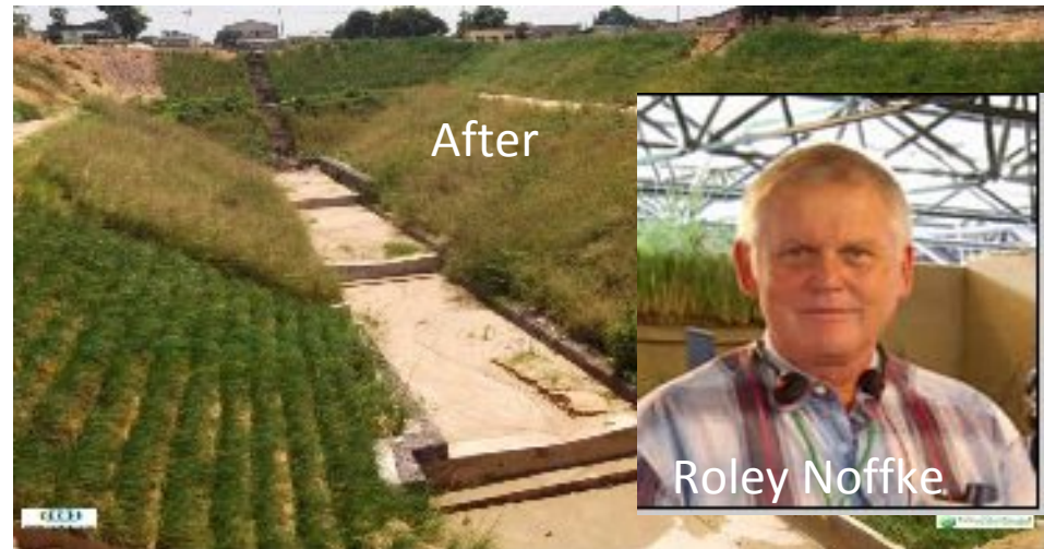
Urban gully rehab - contracted
