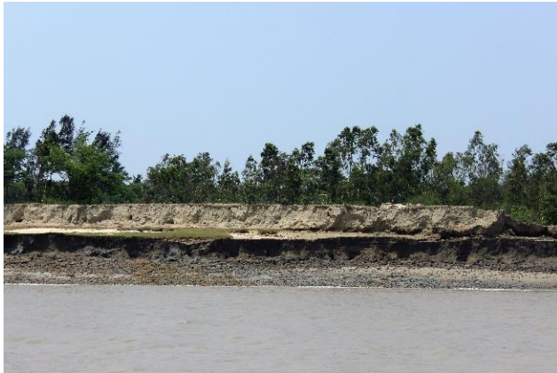
Eroded Protection dike on GHORAMARA Island
