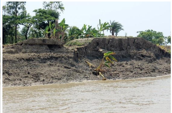
Eroded Protection dike on GHORAMARA Island
