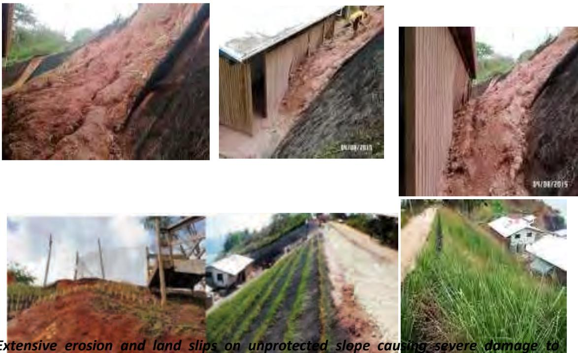
***Extensive erosion and land slips on unprotected slope causing severe damage to buildings prompted authority to adopt Vetiver System Technology.***
