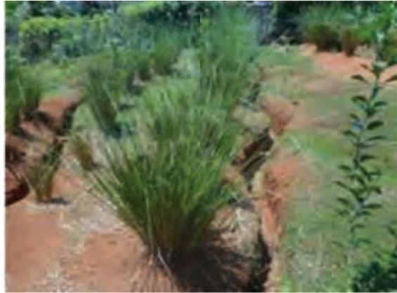
**Picture 21 & 22:** Vetiver planted in front of drains which were dug initially to reduce velocity of water to control soil erosion on hill top.
