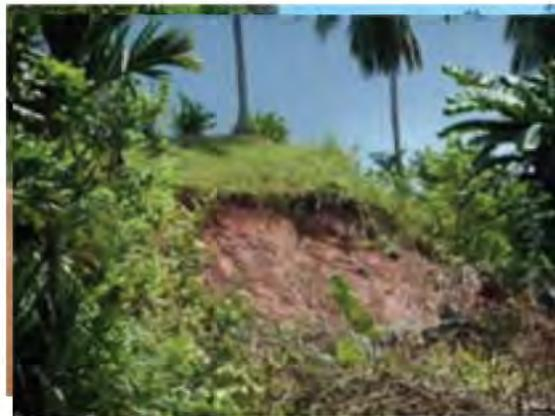
**Picture 42 & 45:** Slope failures like this are common sites for the township which poses immediate danger. Two houses were buried by this slip in January. Slope stabilization of these sites will serve multipurpose objectives - land slip protection, garden erosion control, soil fertility improvement.
