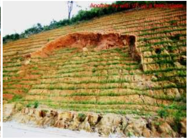
Vetiver planting on a fill batter
