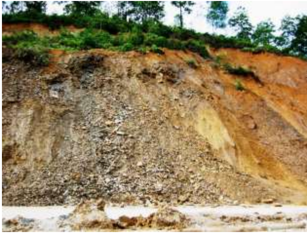
Horrific erosion on a cut batter
