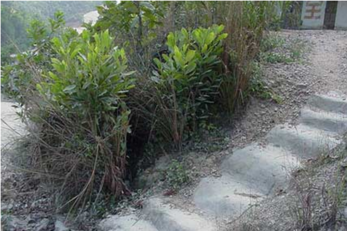
The same site three years after vetiver had been planted -- vetiver well established and native plants are developing. (cross sectional view).
