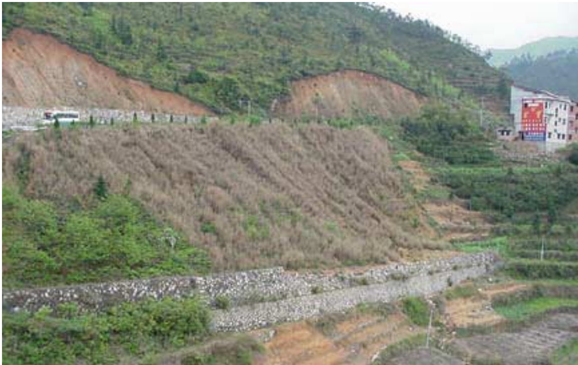
Highway stabilized with vetiver. This is a very large and steep slope with hard measures at the base only. Prior to the planting of vetiver the rock wall at the base of the slope was regularly breached. Note how there has been rilling, but now the slope is stable.
