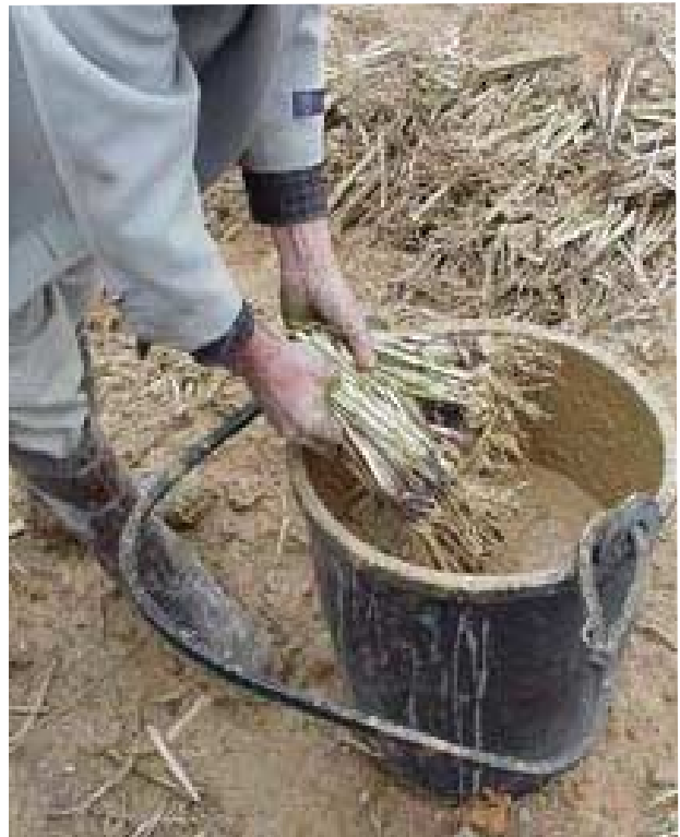
Vetiver slips dipped in a mud slurry prior to planting at the highway site
