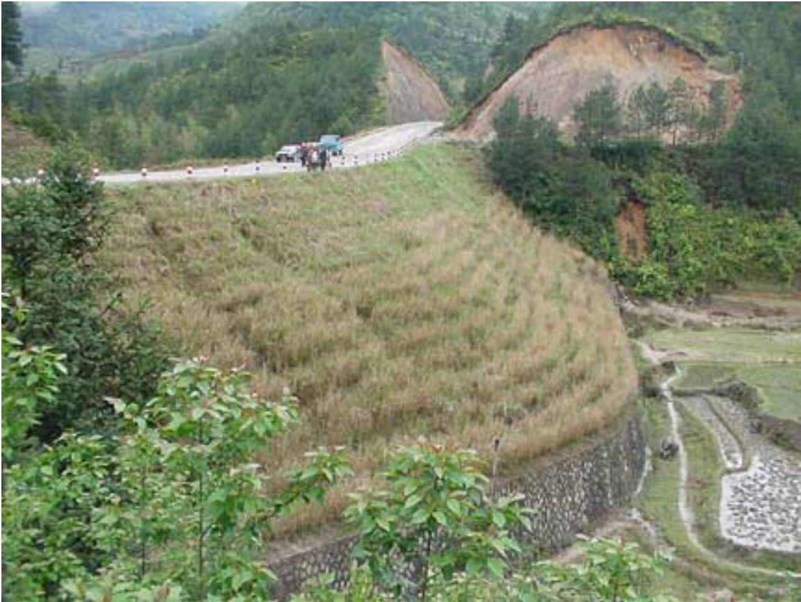
Provincial highway stabilized with vetiver. Planted April 2001. Note the combination of “hard” and “soft” measures. The top few rows of vetiver have been recently cut. There was some rilling on the left hand side but the slope has now stabilized. There remains a management problem.
