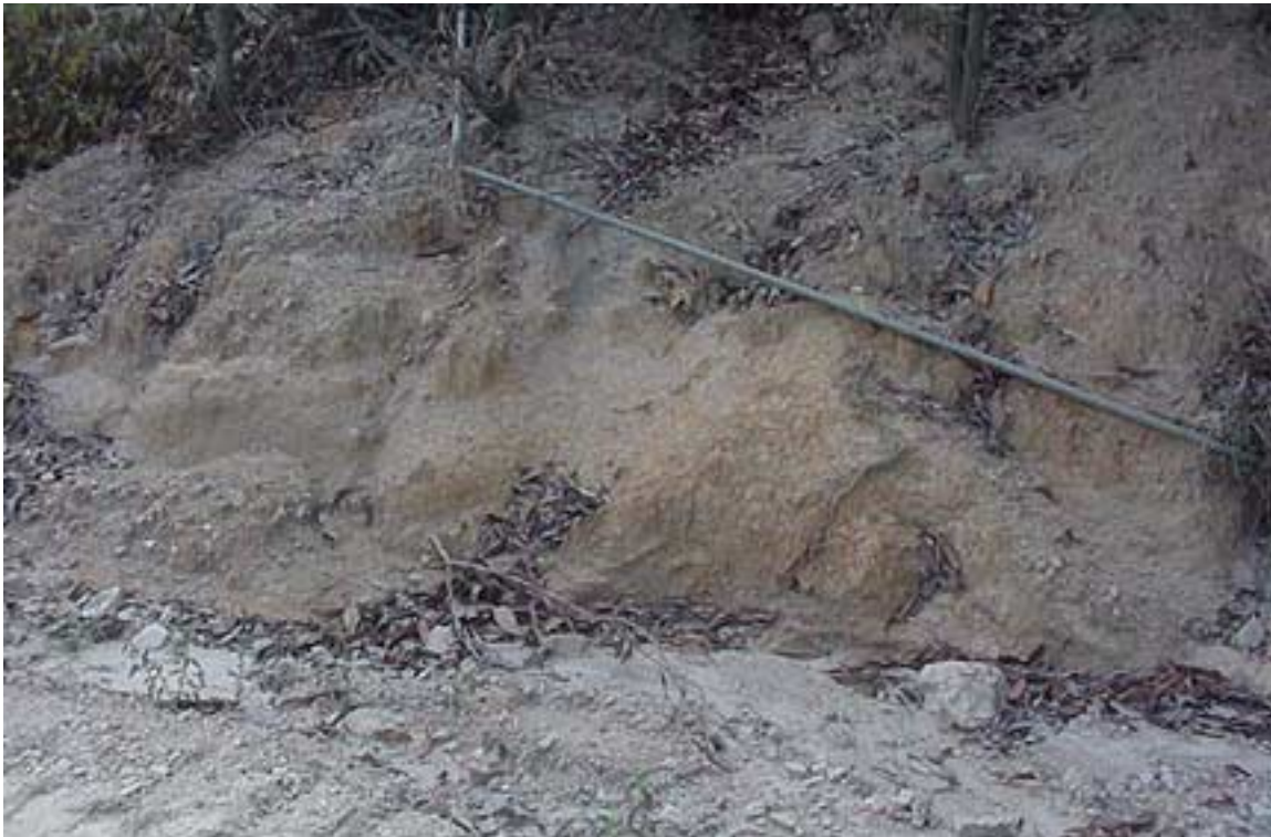
This image is of the slope below an oil storage shed in the quarry. No plants would grow here.
