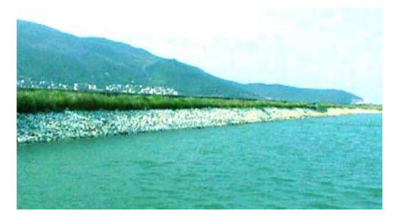
Figure 16-24b. The vetiver hedge (the same as in Figure 16-24a) is not affected by seawater.
