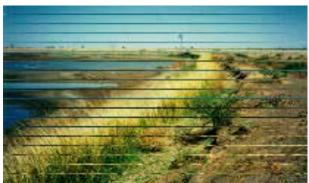
Figure 16-24a. On China's Pintang Island, vetiver hedges protect the sea wall around a fish farm. This hedge has protected the wall from the effects of a typhoon that wrecked the unprotected walls in other parts of the farm. The roots of the vetiver extend down to the wall's base and protect it from the internal runoff from the land behind.
