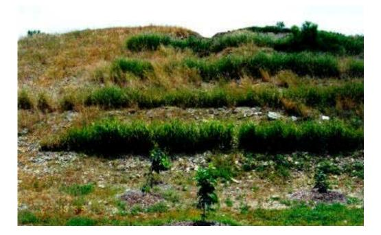
Figure 16-23a. In Queensland, Australia's outback, workers plant a vetiver hedge at the water line (green ink line) to prevent lap erosion from destroying this vital source of water storage and to prevent further silting.
