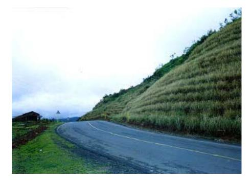
Figure 16-20b. This road in Malaysia, that suffered severe collapse was eventually stabilized using vetiver hedges, and no further problems have occurred where the hedges were well-established. Nonetheless, engineers were still skeptical, asking for proof.
