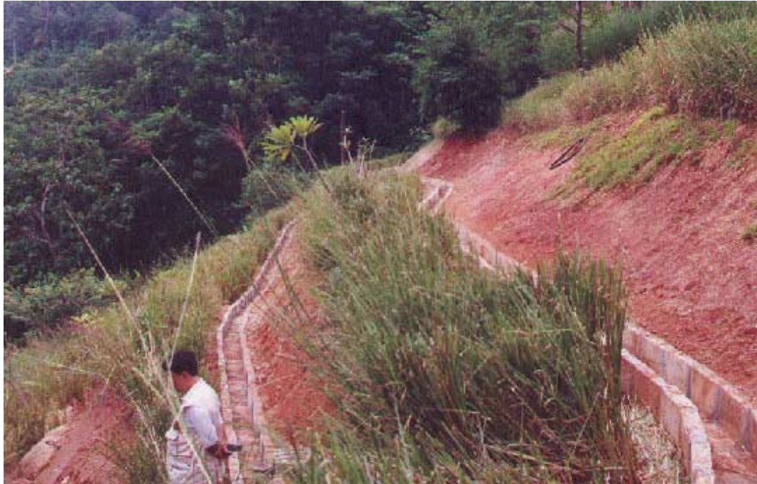
Fig. 15 Combination of Vetiver and mechanical measures in road bank stabilization; Chiang Mai, 1999.
