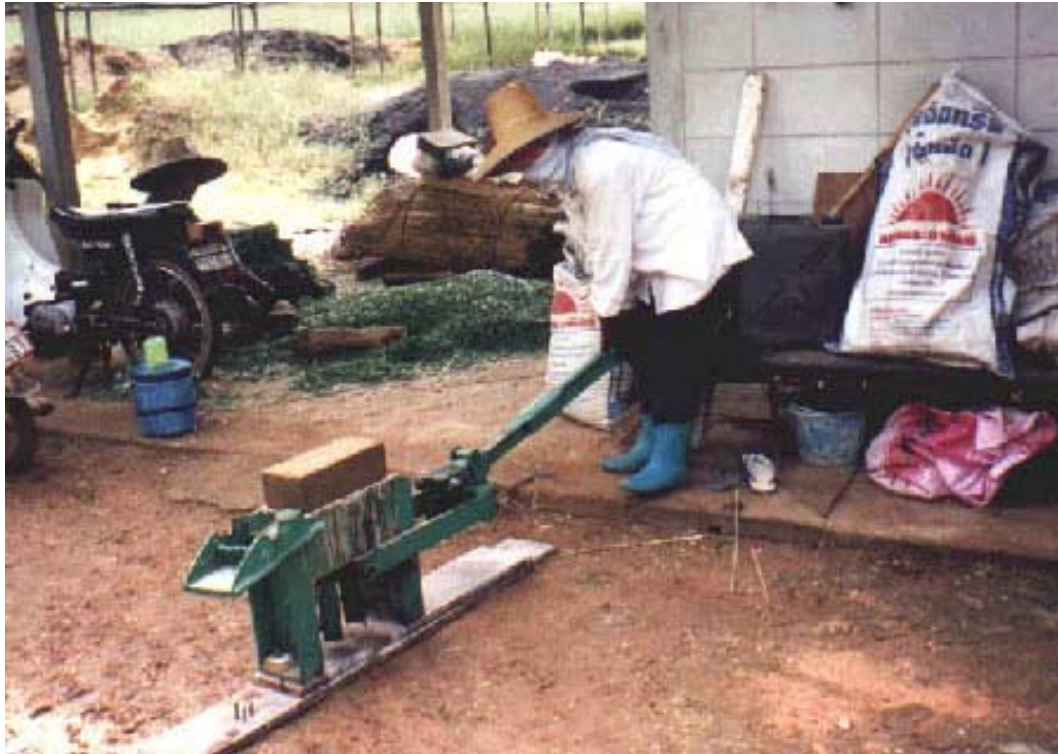
Fig. 20 Vetiver soil-cement brick developed for native clay cottage improvement. The wall bearing load reduces the cost of household construction; Ratchaburi Land Development Station, DLD Region 10, 1999.
