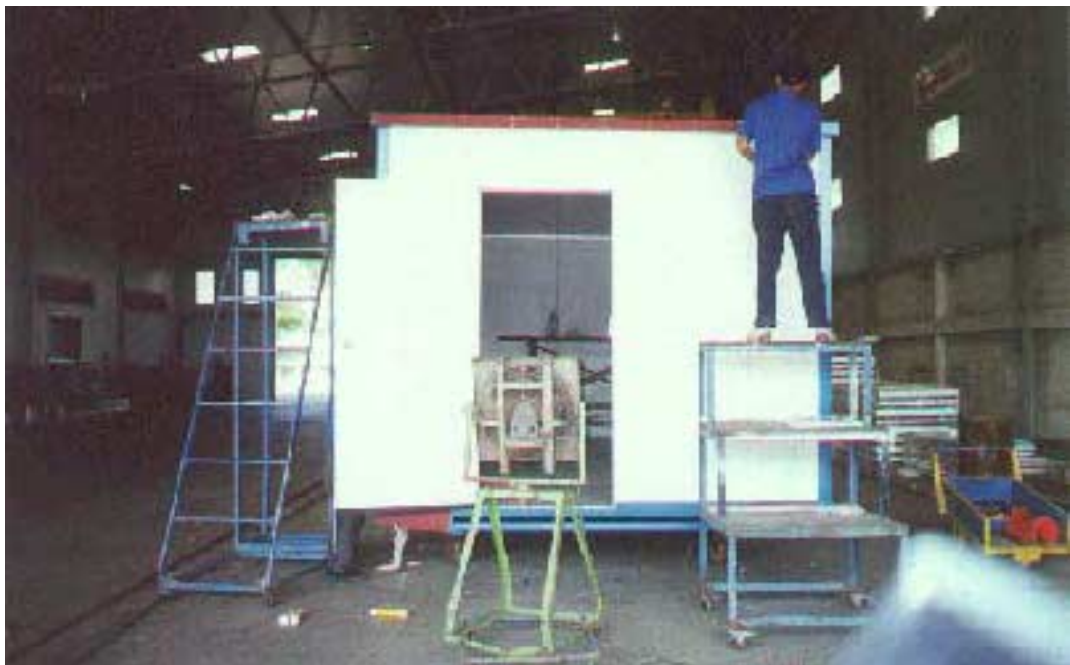
Fig. 27 A cabin using Vetiver thermal insulator panels under construction for exposure testing; Great Wall Insulator Co, Ltd., Patumtani, 1999.
