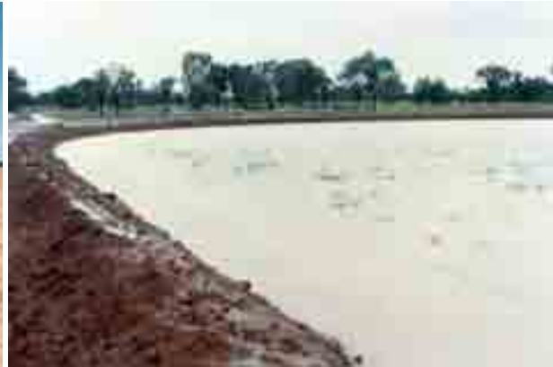
Catching rain water to 20-30cm depth
