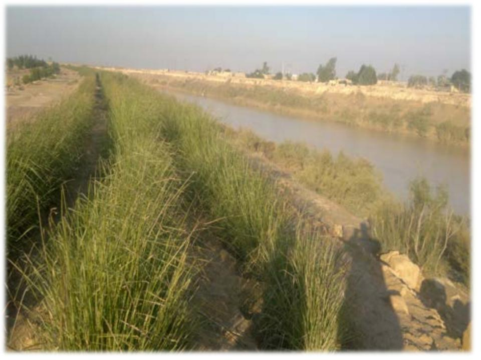
In the north of Iran ( Humidity province) Gilan province for slope stabilization and protection of both sides of agricultural irrigation channel. Along water way channel there was erosion, land slid and crash mass of the soil in to the channel and made different problems.
