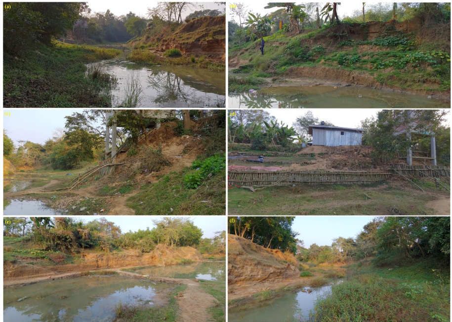
Fig. 8 Views of the unprotected left and right bank of the Ketia River at Gholsai village in January, 2020, with both banks being markedly eroded in the preceding summer monsoonal flows, showing a , c , d the eroded section on the concave right bank upstream of the Vetiver-protected section, even though attempts had been made to protect a portion with just bamboo stakes, but bereft of the Vetiver coverage b rotational bank slumping on the left bank, and e , f sections suffering marked erosion even on the inner left bank, while the opposite Vetiver-protect right bank shows much more stability
