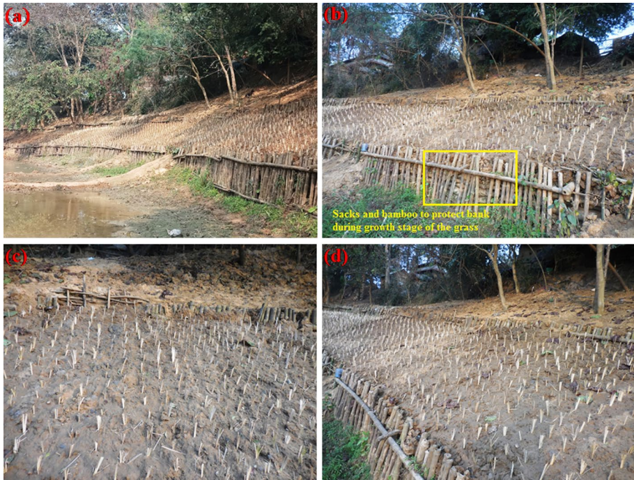
Fig. 5 Recently transplanted Vetiver saplings at Gholsai village ( 22^{\circ} 36' 30'' N, 87^{\circ} 37' 52'' E)—with a , c , and d showing different views, and with b denoting the sand-filled sacks and bamboo cuttings placed on the toe slope and along the bottom of the riverbank in order to protect it while the Vetiver grass grows fully
