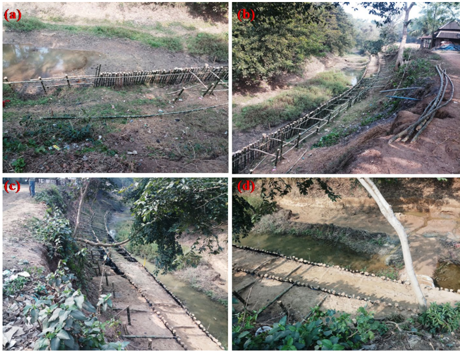
Fig. 3 Reach of the Ketia River at Shyampur village ( 22^{\circ} 36' 36'' N, 87^{\circ} 37' 33'' E), Ghatal Block, being prepared for planting the Vetiver buffer, a driving in of bamboo stakes, b aligning bamboo geogrids with bank geometry, c earth filling of the bamboo grids, and d a completed slope segment ready for transplantation
