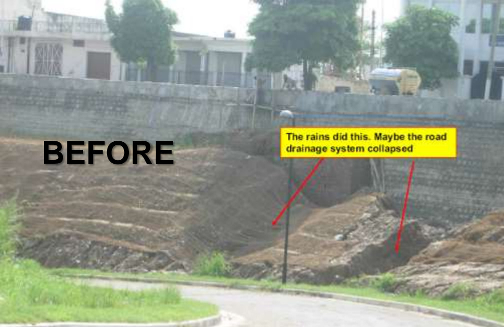
The earth has given way from under the geo-textile
