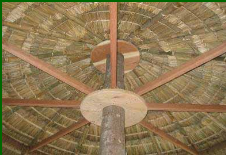
Underneath view of thatching
