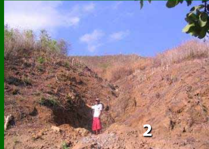
After clearing bushes & grasses
