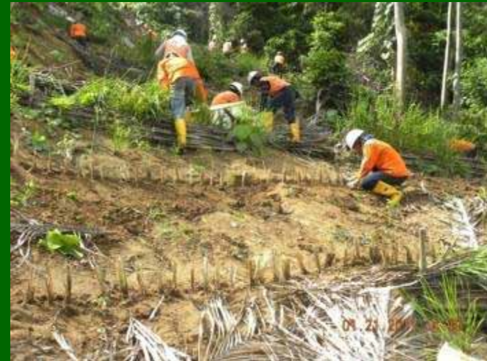
Planting vetiver on steep 400m slopes around the Base Transceiver System (BTS) & new power lines
