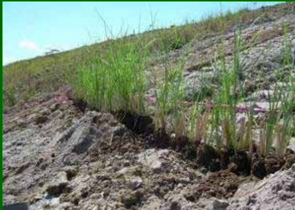
April 2010: Planted 2,200 vetiver slips in polybags for 1 month prior to planting on tailngs slopes
