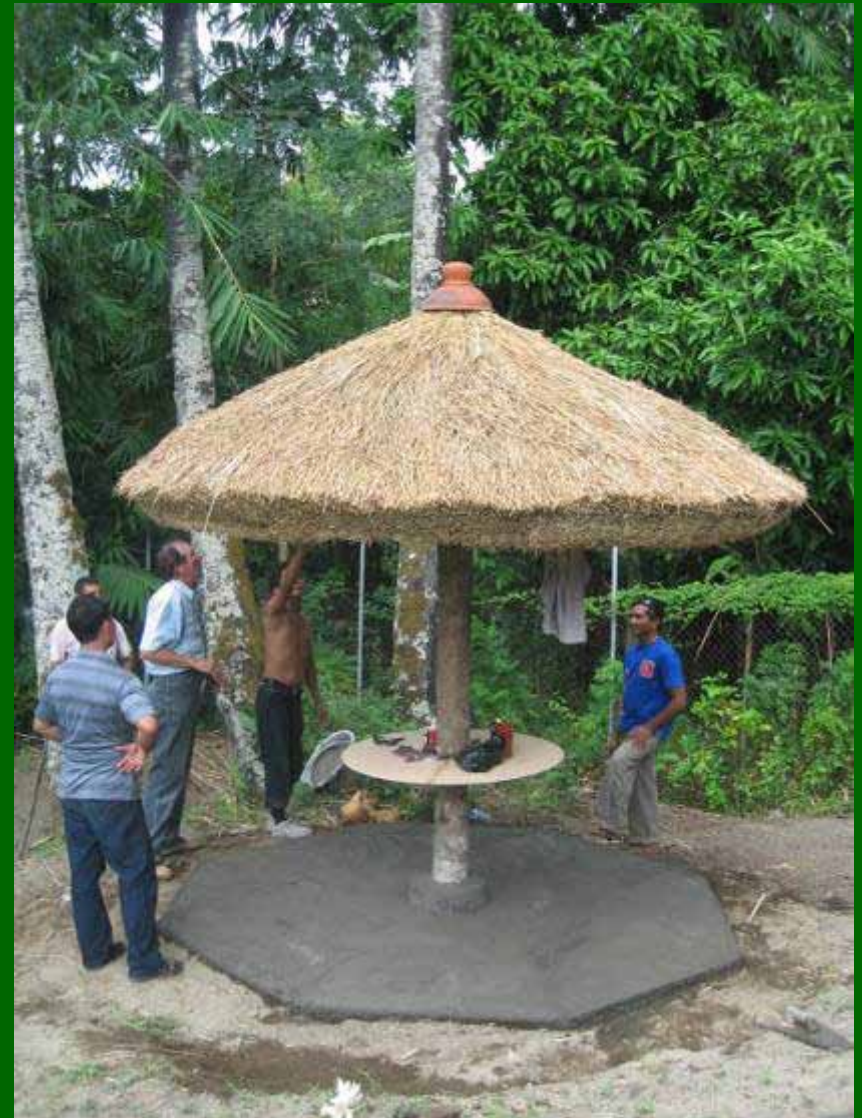
Completed recreation area vetiver "umbrella"
