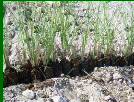
Vetiver planted with 2 meter vertical interval, row distance: 5,4 meter and slips distance : 15 – 20 cm
