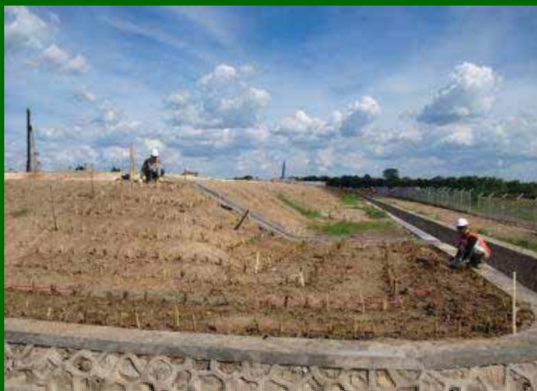
Planting Vetiver on platform corner slopes
