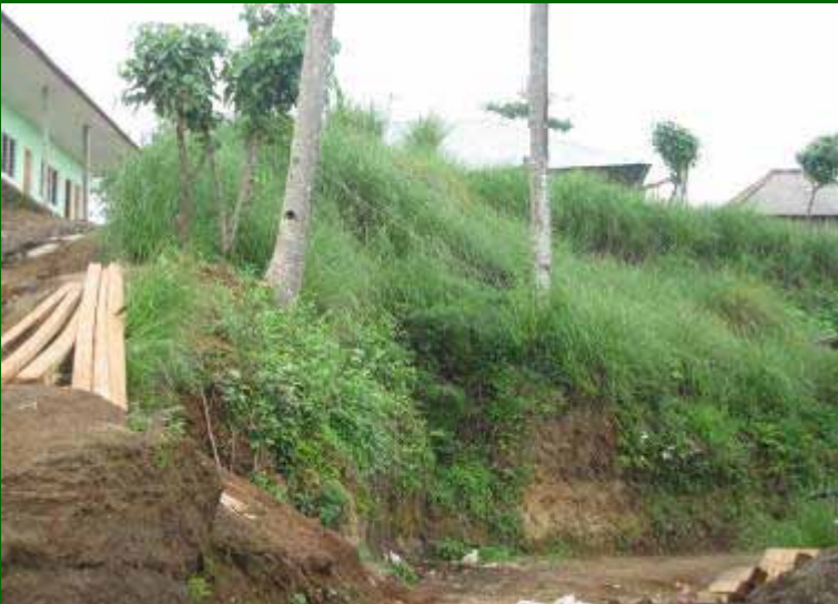
Vetiver stabilizes Steep embankments in front of school
