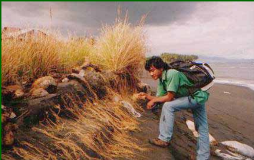
Fierce waves erode steep sand slopes – Vetiver survives
