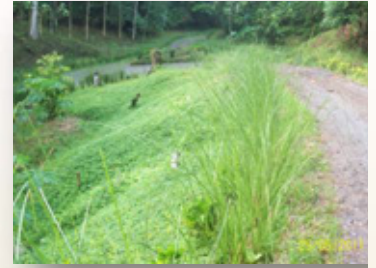
Plantation office road batter stabilized (Kimbe PNG)
