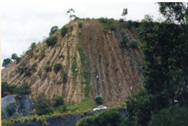
Before and after vetiver planting on a old coal tailings dump in Queensland. Very steep and highly erodible old dump (left) Vetiver planted to control erosion and rehabilitation
