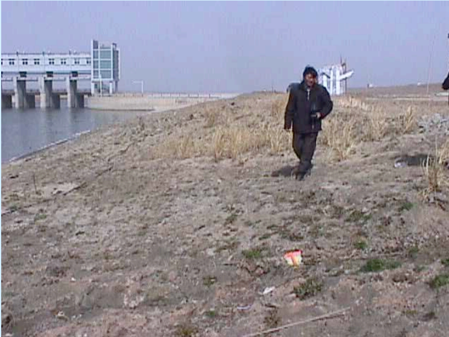
Failure by low temperature
