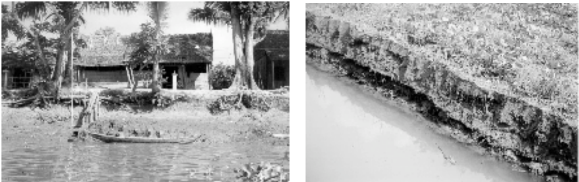
Photo 2 Left, Erosion on the bank of a tributary. Right, Erosion on the bank of the Mekong
