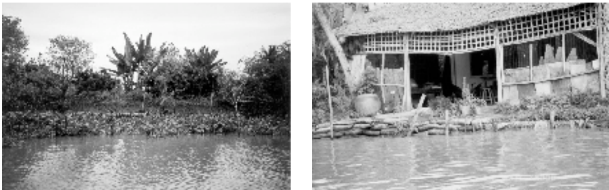
Photo 3 Left, Vegetative method with water hyacinth. Right, engineering method with sand bags
