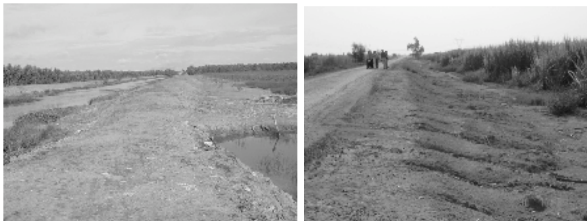
Photo 1 Severe erosion on canal and rural road on Acid Sulfate soil
