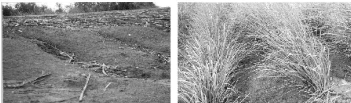
Photo 9 Soil loss was reduced from 400-750 tons/ha to only 50-100 tons/ha on the channel embankment
