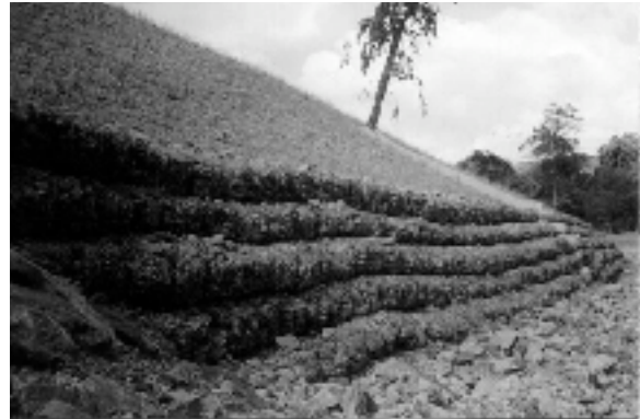
Fig. 13 VS is associate with gabion wall in the rehabilitation work on Highway Route No. 1451: Sec. Adj. to Phattalung Highway District's Area – JRT. Highway No. 403
