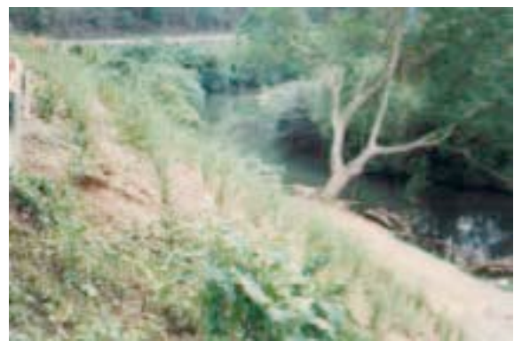
Fig.9 Stabilization with vetiver along the stream bank on Highway Route No.107: Ban Pingkoke – Saphan Huai Tai.
