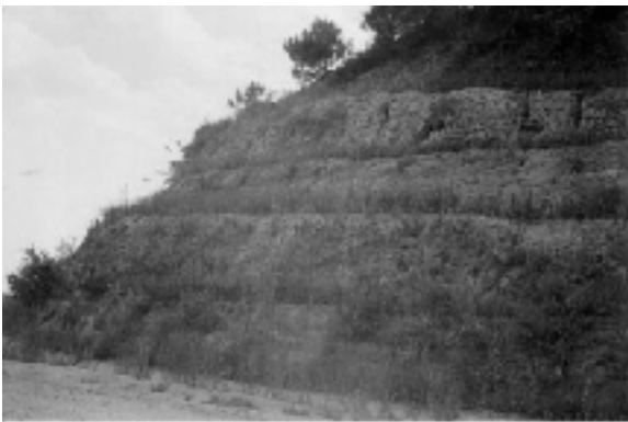
Fig. 5 Highway cut slope was stabilized with vetiver on Highway
