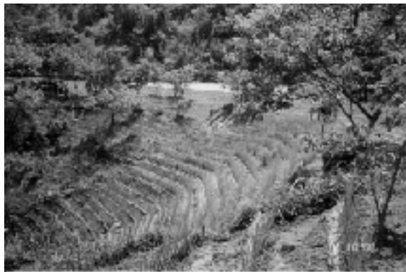
Fig. 6 Highway embankment was stabilized with vetiver on Highway Route No. 1149
