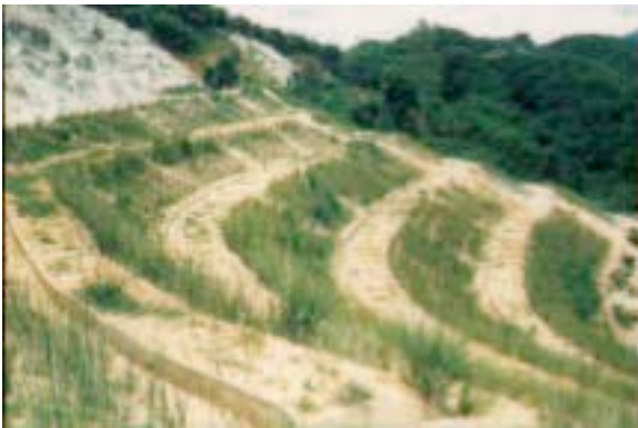
Fig. 8 High embankment was stabilized with vetiver coupled with surface drainage systems in the rehabilitation on Highway Route No.109: Fang – Tha Thon
