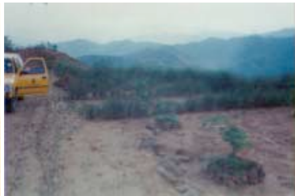
Fig. 11 Vetiver planting on highway shoulder should to slow down runoff longitudinal
