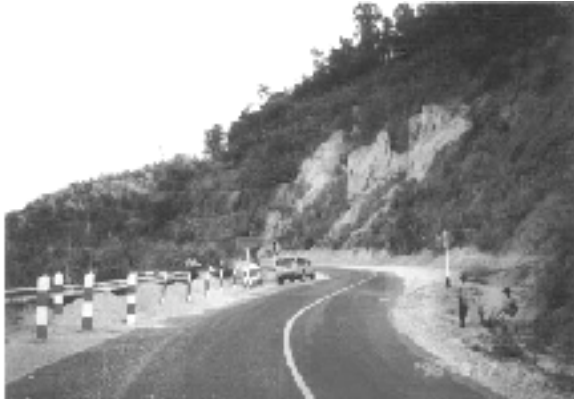
Fig. 1 The strongly erosion on granitic soil back slope, sediments fill up ditch and damage embankment slopes
