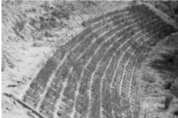
Fig. 12 VS is applied with concrete square grid slope protection in the rehabilitation work on Route No. 108: Hot – Mae Sariang
