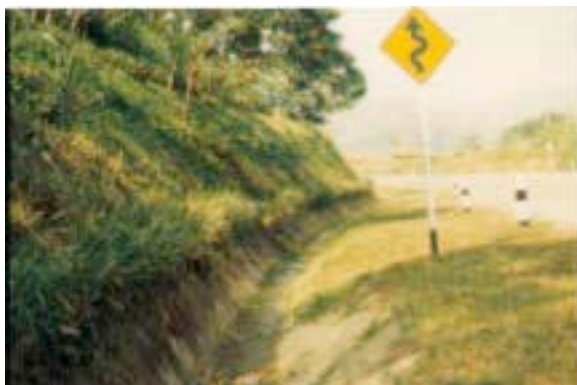
Fig. 10 Vetiver planting at the side ditch lining
