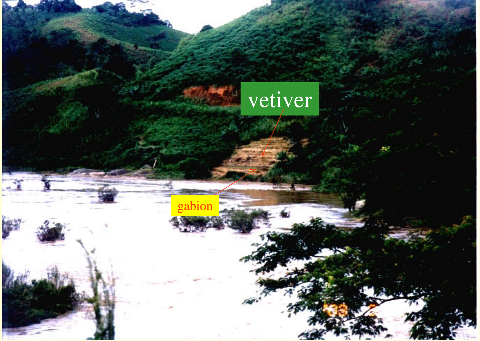
Vetiver w/ gabion by riverbank
