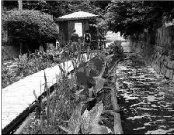
Photo 1 Hydroponic treatment of sewage with other plants
