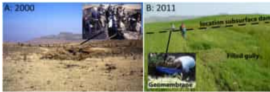
Figure 7. After the introduction of the subsurface dam at the gully head in vertisol in Khunale in 2000 (A), the gully was stabilised and filled (B), and the geomembrane dam remained intact. Panel (A) was taken in the dry season and panel (B) in the rainy season. This figure is available in colour online at wileyonlinelibrary.com/journal/ldr .
