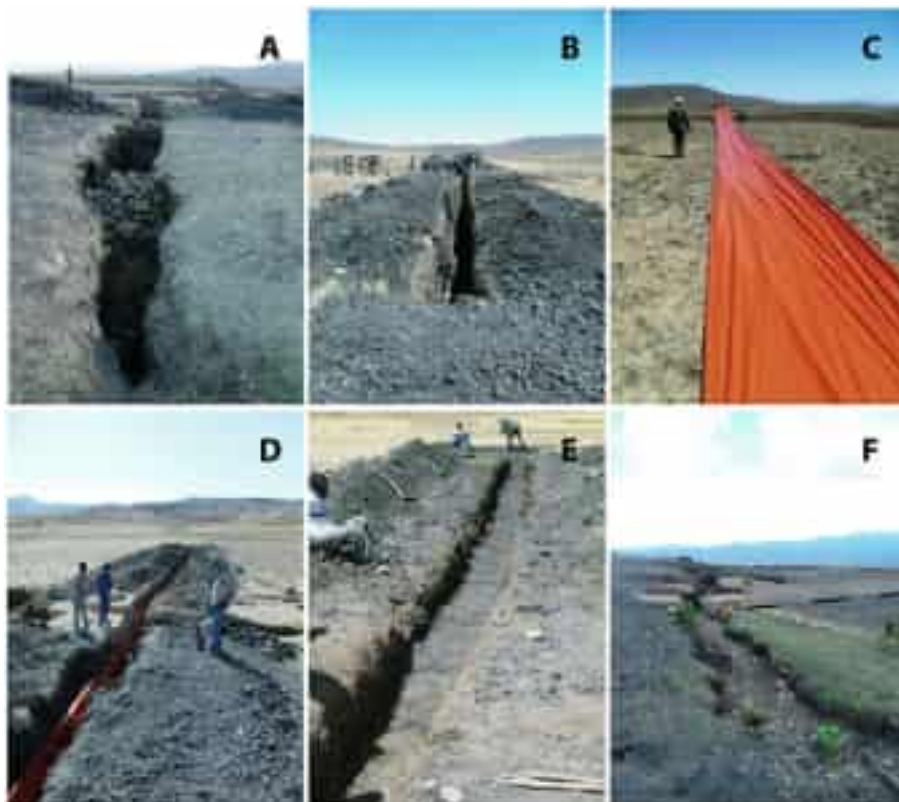
Figure 6. Introducing a subsurface geomembrane dam to stabilise gully heads in a vertisol area in May Ba'ati, Ethiopia. (A) Reinforcement of the headcut with a gabion check dam, (B) digging of a 25 m long and ca 2.3 m deep trench in the intergully area at both sides of the gabion check dam, perpendicular to the gully, (C) the geomembrane (bought from a nearby shop), and (D) introducing the geomembrane into the trench. The upper 0.3 m of the soil profile was not dammed to allow tillage and cropping, (E) filled trench. (F) View on the gully head 1 year after installing the subsurface dam. Upslope from the dashed line, which indicates the position of the subsurface dam, the grass is greener and soil moisture is better as compared with the lower side of the dam. This figure is available in colour online at wileyonlinelibrary.com/journal/ldr .
