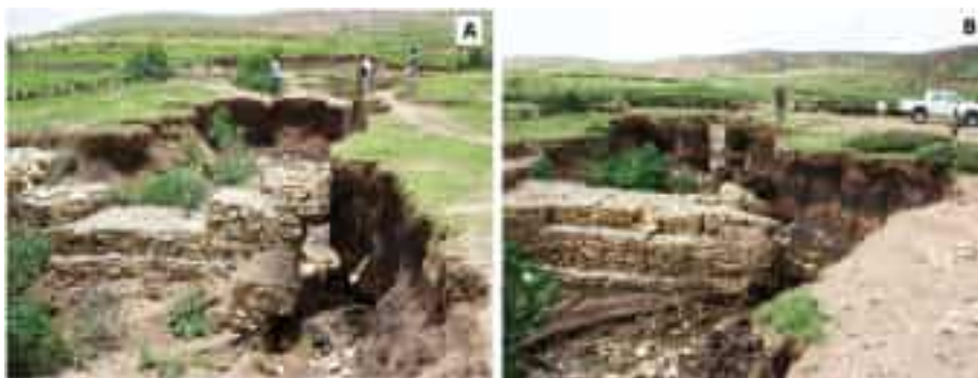
Figure 2. (A) Because of soil piping in a vertisol lens near the check dam (white arrow), the latter was bypassed in 2011. (B) To counter this, the check dams were re-enforced in early 2012. Soil piping did, however, again cause bypassing of the check dam and the expansion of the gully in the adjacent land (intergully area; May Ba'ati, Ethiopia). This figure is available in colour online at wileyonlinelibrary.com/journal/ldr .
