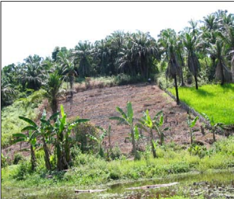
Photo 1: Typical unprotected and eroding slope
