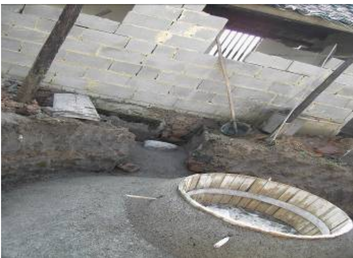
A bio-gas tank was finished
