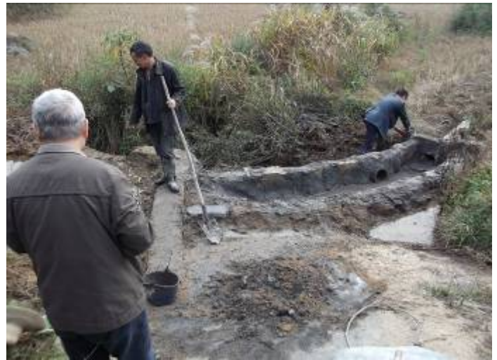
Reconstruct ditches and install pipes
