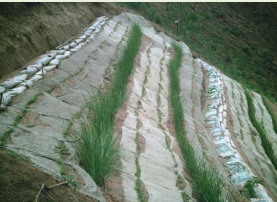
Planting on contour lines ay 1m Vertical Interval
