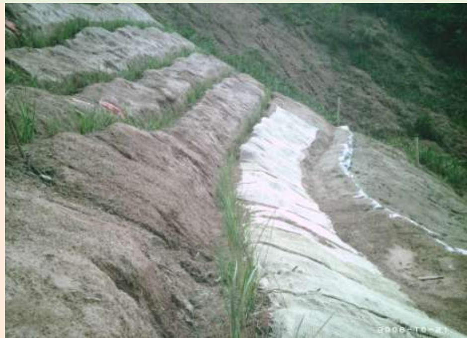
Planting on contour lines ay 1m Vertical Interval
