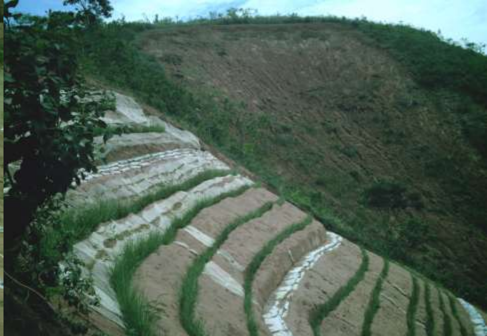
Planting on contour lines ay 1m Vertical Interval
