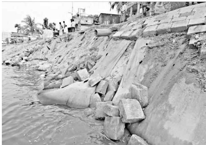
Figure 2.7: Poor performance of CC blocks at Keraniganj Beribadh site (Source: Prothom Alo, dt: 04.04.2011)
