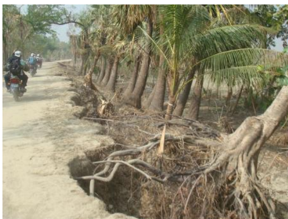
Figure 2.4: Failure of embankment due to overturning or uprooting of trees during cyclone (Mohammad Shariful Islam, BUET)
