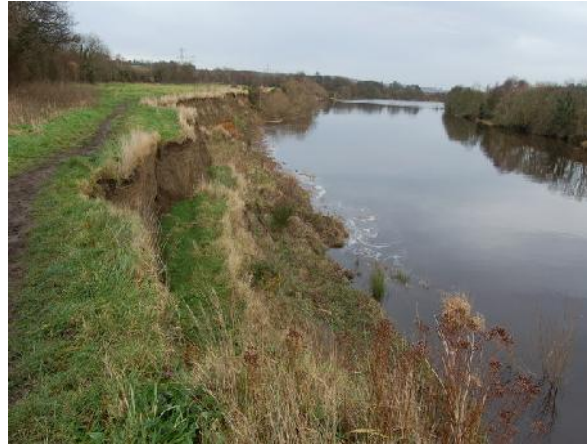
Figure 2.3: Photograph showing failure of embankments due to turbulent water currents (Wikimedia Commons, 2010)
