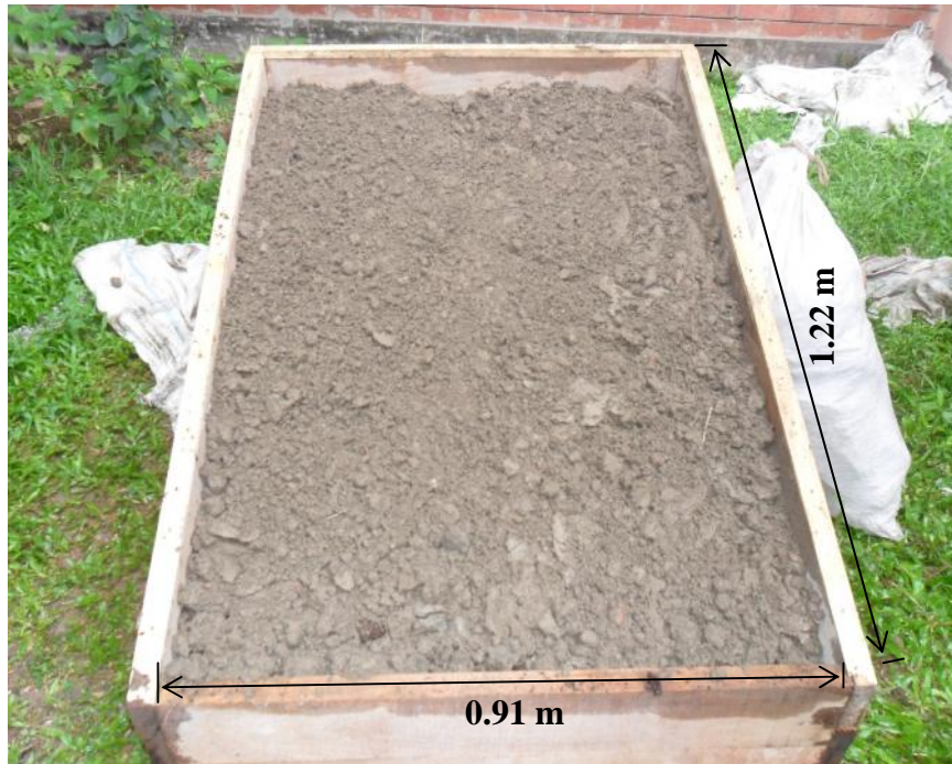
Figure 3.10: Preparation of the slope
