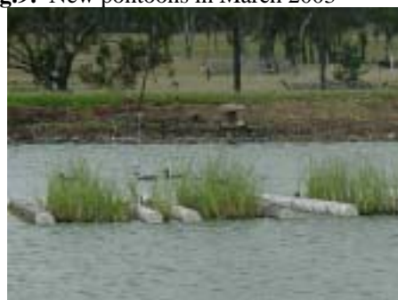
Fig.9: New pontoons in March 2003
