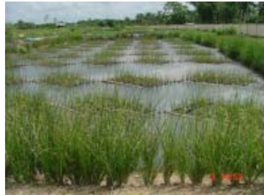
Fig.6: Vetiver pontoons treating a piggery effluent pond in Vietnam
