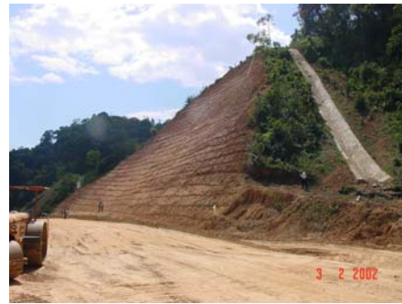
Spring Pass demonstration site, showing the steep slope and no on-slope drainage bench
