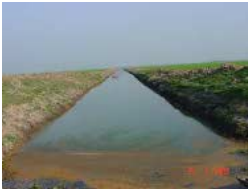
The demonstration site on a submergible dyke at Tri Ton.
