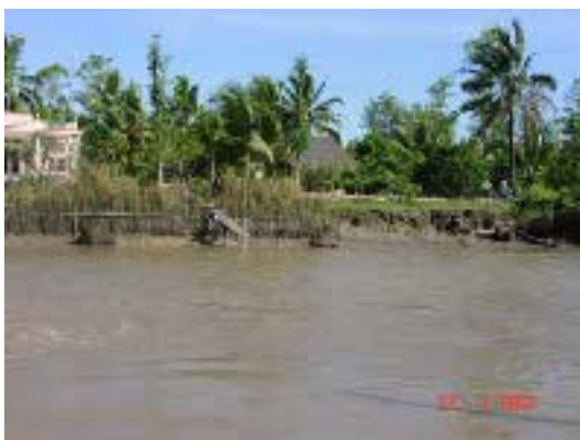
Site for comparison between vetiver and Phragmites on this canal bank
