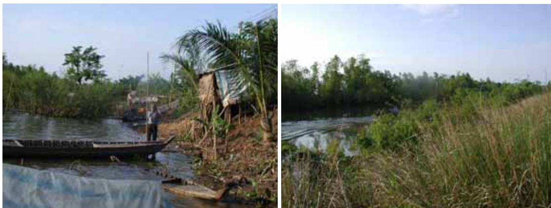
Left: Unprotected dike during flood and Right: Dike protected by vetiver
