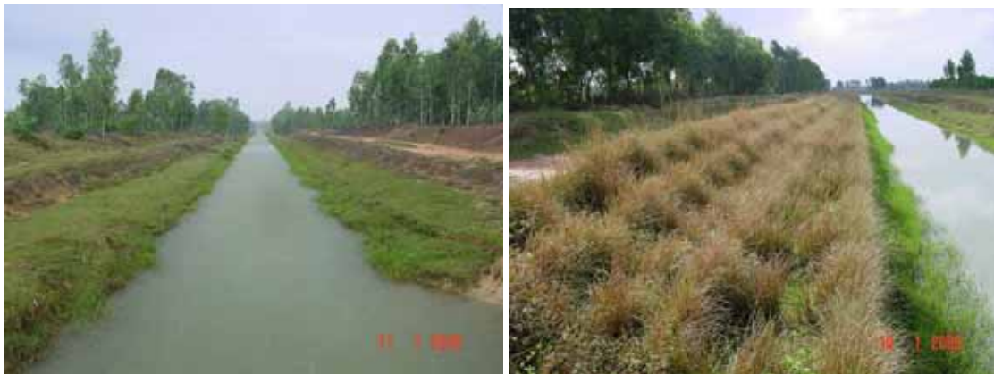
A drainage channels before and after VS protection
