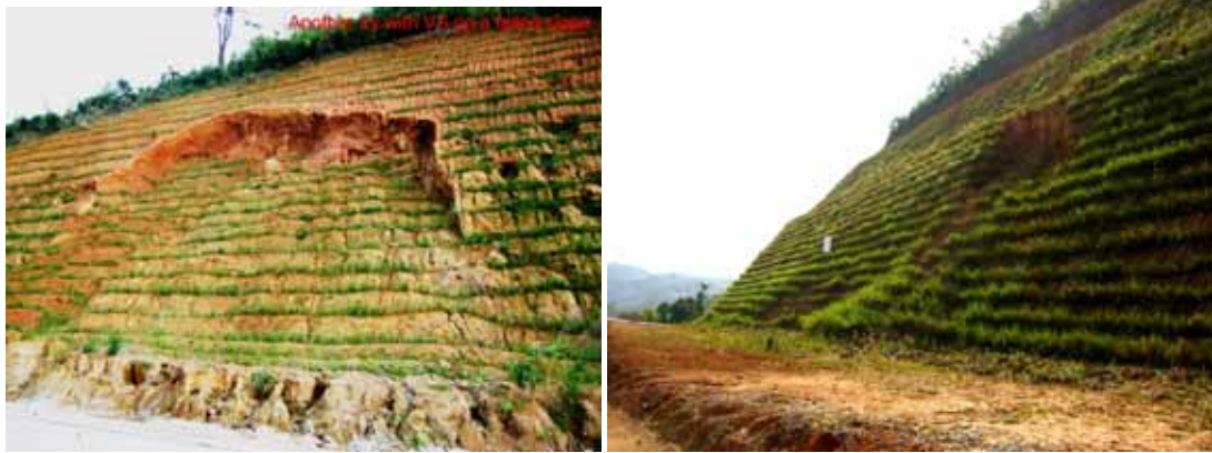
Left: Vetiver should not be planted on this high slope (55m vertical drop) without benching, but so far so good as this batter is on a less erodible soil. Right: A well designed and planted batter with benches and on erodible soil among more stable rock surface
