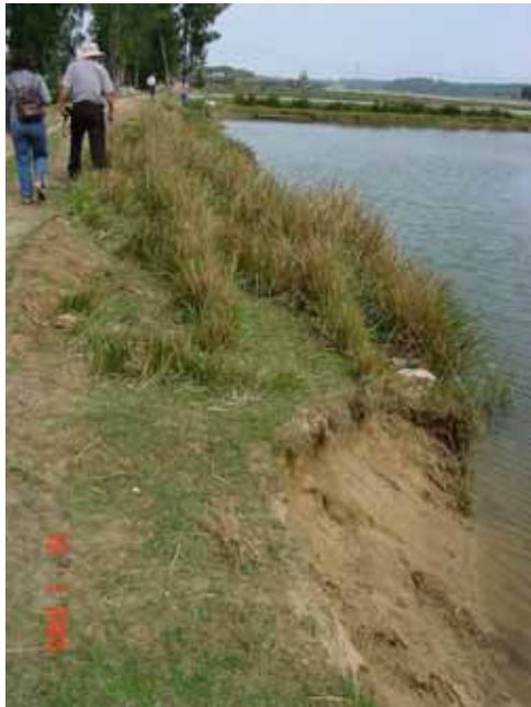
An estuarine dike with and without VS protection (left), the mangrove fern on the water edge below the vetiver hedge
