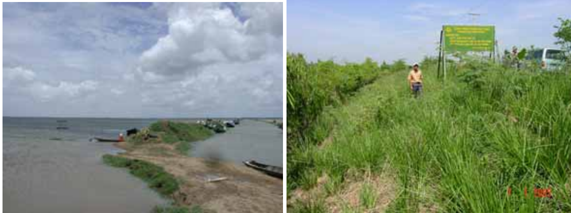
A broken dike during flood and the batter of the 17km long dike protected by the VS
