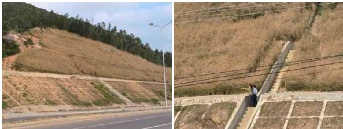
Vetiver has successfully stabilized the steep and rocky part of this batter, while the more expensive hard structure was used on a gentler lower slope
