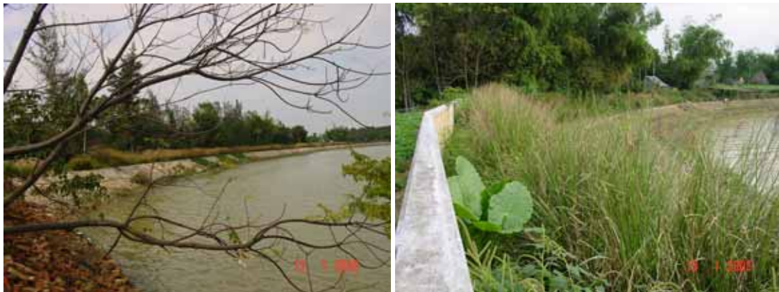
VS in combination with rock paving on a large riverbank at Da Nang (left) and the bank on the bend of the river was stabilized by vetiver alone
