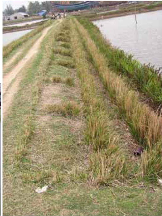
An estuarine dike before and after VS protection, note the mangrove fern on the water edge below the vetiver hedge
