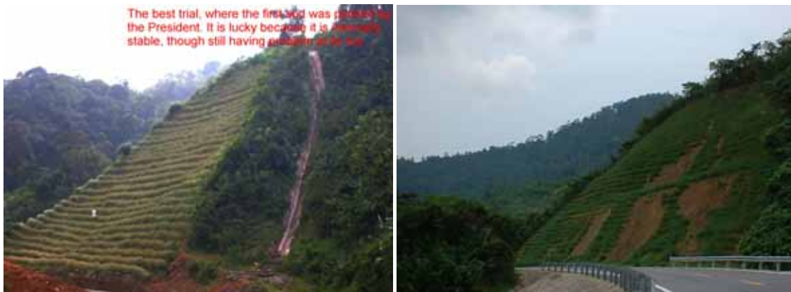
Left: Vetiver should not be planted on this high slope (55m vertical drop) without benching, but so far so good as this batter is on a less erodible soil. Right: A well designed and planted batter with benches and on erodible soil among more stable rock surface
