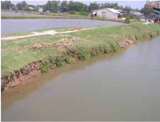
An estuarine dike with and without VS protection (left), the mangrove fern on the water edge below the vetiver hedge
