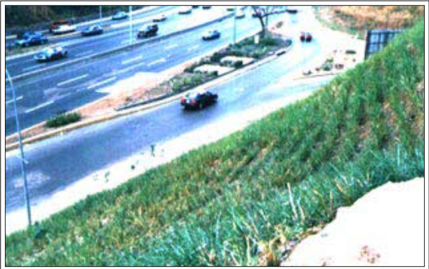
VENEZUELA: Stabilization of steep highway cut in Caracas using VS. VS should be used to rehab Caracas Flood Damage.
