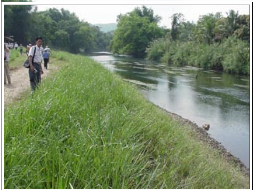
Thailand. Vetiver and water. A river levee stabilized with vetiver grass. The stabilization was fully effective, and when over topped by flooding was completely stable. Photo Credit: Dick Grimshaw.
