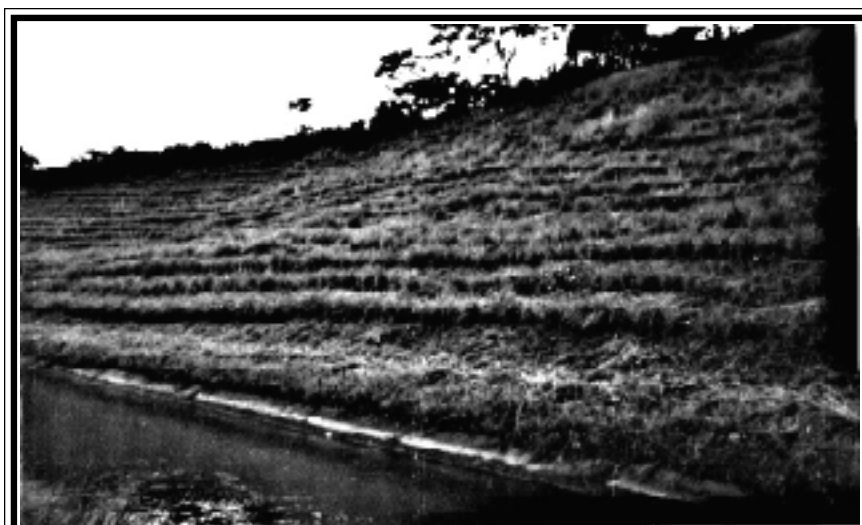
Canal cut at Manupali, Philippines, stabilized with vetiver grass hedge rows
