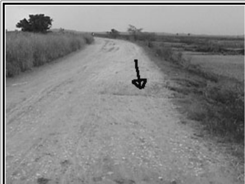
This road on an irrigated rice project at Marovayi, near Mahajangais fully protected on the left hand side with vetiver grass. On the right there is no vetiver protection and rilling is taking place on the road (by arrow)
