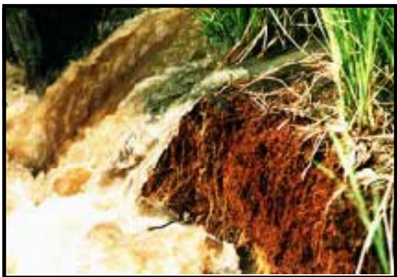
Above. This section is being cut by water flow. Even so vetiver roots provide mattress to retard rate of cut. Next year this should be fully stabilized.
