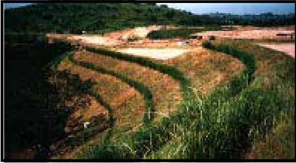
Above: Buiding site in Natal, South Africa, stabilized with vetiver hedgerows. Contractor: Tony Tantum. Photo Credit: Paul Truong
