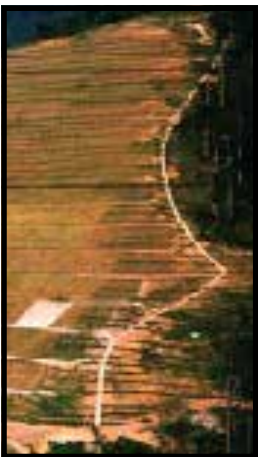
Above: Malaysian Highway Stabilisation, Left: Vetiver grass stabilized the upper half of this 180 m VI slope. Lower half, conventional engineering technology. Right: vetiver stabilizes the weak area at interface with drainage ladder. Contractor: Diti Hengchaovanich. Photo Credit: Paul Truong
