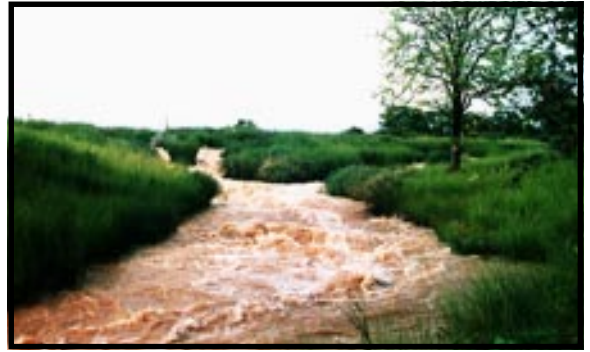
10,000 lt per sec emerging in channel at bottom of spillway. Fully protected with vetiver hedgerows
