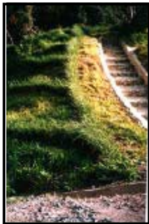
Above: Malaysian Highway Stabilisation, Left: Vetiver grass stabilized the upper half of this 180 m VI slope. Lower half, conventional engineering technology. Right: vetiver stabilizes the weak area at interface with drainage ladder. Contractor: Diti Hengchaovanich. Photo Credit: Paul Truong
