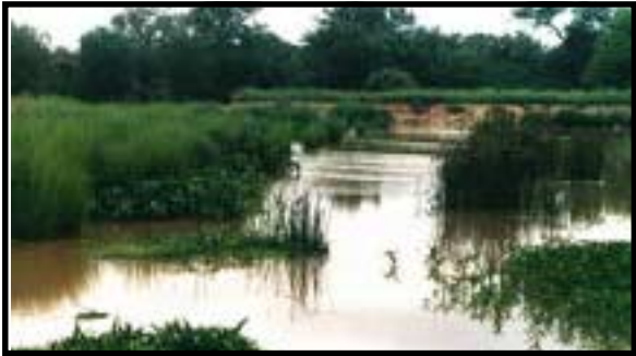
Spilling sill of 80m wide spillway, protected by vetiver on spillway side at left.
