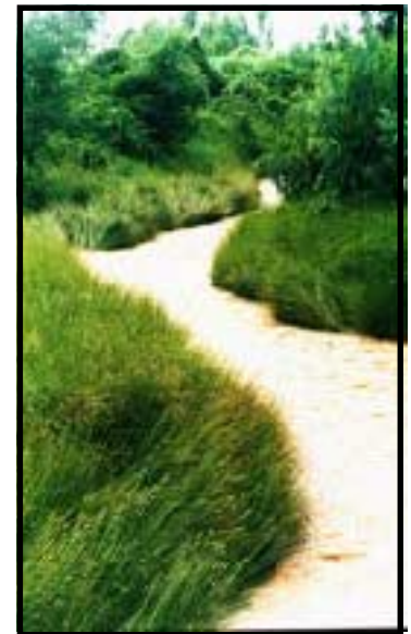
Above: 12 km river, fully protected by vetiver grass hedgerow, that carries some 10,000lt per sec from one reservoir to another down stream. River banks now totally stable.
