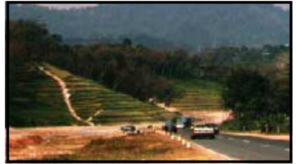
Above: Malaysian Highway (general view) stabilized with vetiver hedgerows. Contractor: Diti Hengchaovanich. Photo Credit: Paul Truong
