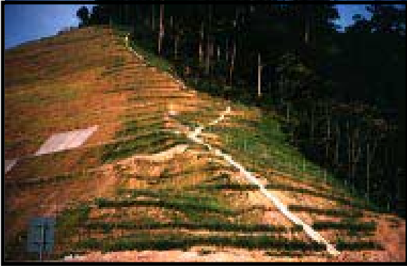
Above: Malaysian Highway Stabilisation, close up of top right scene. The right hand end of this cut received additional reinforcing with vetiver. Contractor: Diti Hengchaovanich. Photo Credit: Paul Truong
