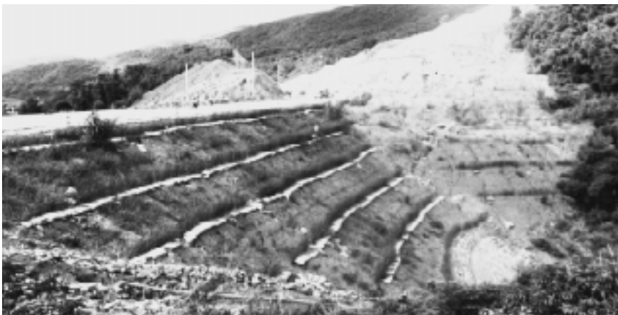
Photo 6 China, Guangdong Province. Highway embankment stabilized with vetiver hedgerows. Photo Credit: Xia Hanping
