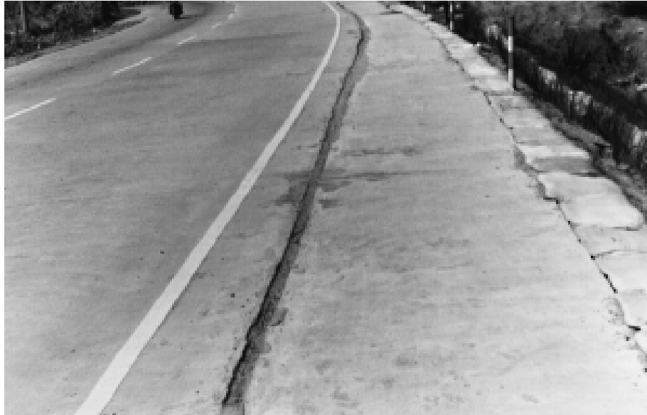
Above: Cracking pavement on a new highway in Guangdong Province due to an unstable embankment. Xia Hanping
