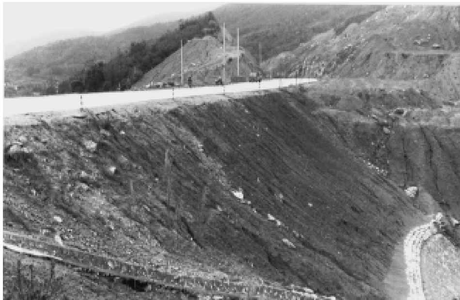
The cracking in the pavement was due to the unprotected embankment shown above. Xia Hanping
