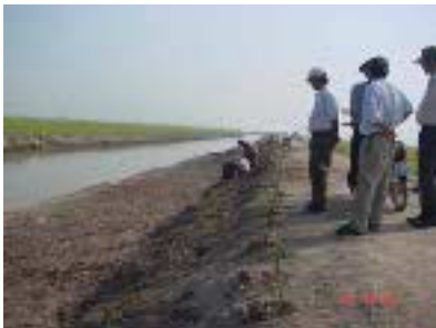
Vetiver being planted on two sides of a dyke at Tri Ton, An Giang province
