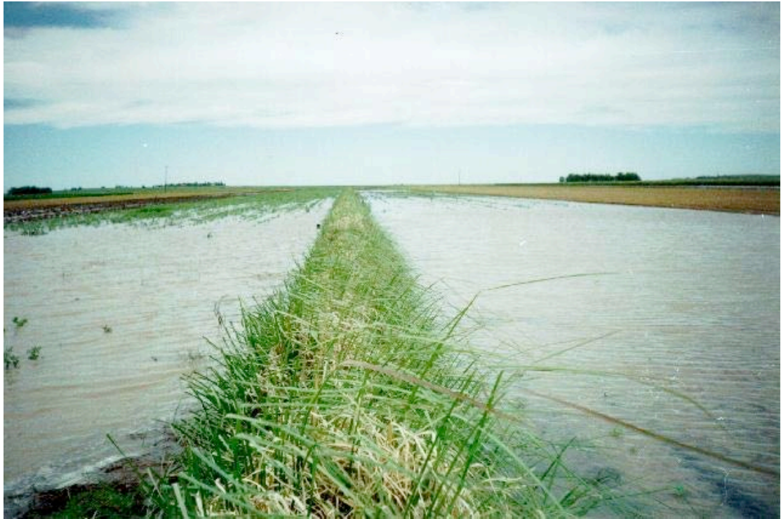
Photo BB47 Shows a vetiver hedge in the Darling Downs Australia containing a massive runoff event, taking the power out of it, the hedge standing up, not breached along its length and protecting crops planted near it. The inundation will not effect the vetiver grass at all, nor the integrity of the hedge.
