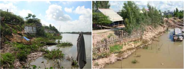
Badly eroded batter and current erosion control measures
