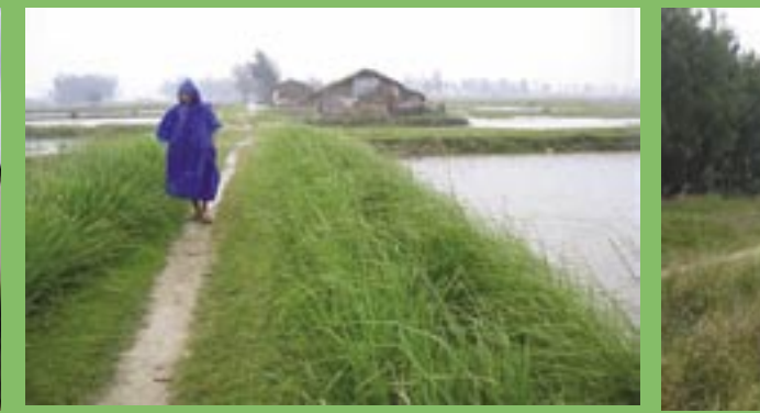
Vietnam - cyclone damage to sea dykes is a major problem. VS has been applied successfully for disaster mitigation
