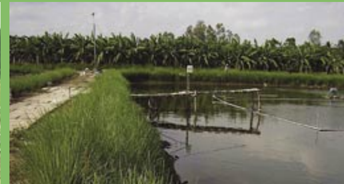
Vietnam - Vetiver is increasingly used to stabilize the banks of fishponds and to purify pond water
