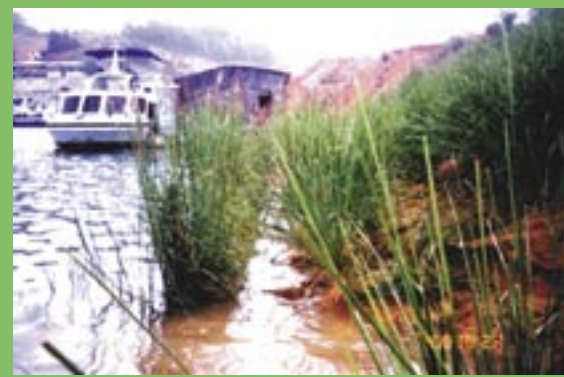
China - partially submerged vetiver grass used to stabilize the draw-down slope of a reservoir in Guangdong Province
