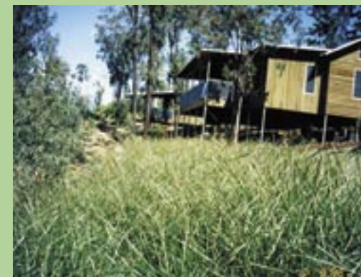
Australia - VS used as a buffer to absorb seeping sewage from this holiday camp site thus reducing runoff and smells
