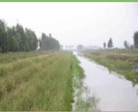
Vietnam - the left hand bank of the canal has been reshaped and stabilized with vetiver, the right bank has yet to be treated.
