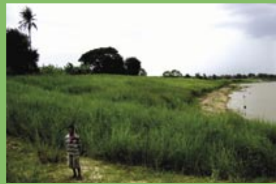
Cambodia - the bank in the previous image has been reshaped and planted with vetiver hedgerows. Very good growth seven months after planting.
