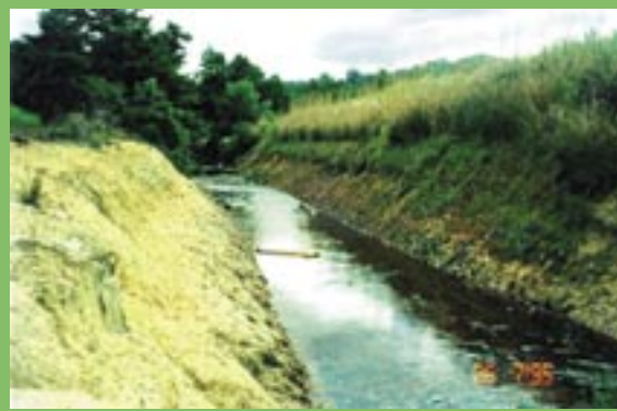
Australia - VS protects the right hand bank of a drain cut through acid sulphate soils of Queensland. Note left hand bank is devoid of any vegetation
