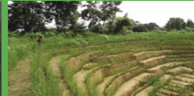
Congo D.R. - huge gullies that destroy urban areas and houses can be rehabilitated and stabilized using the Vetiver System.
