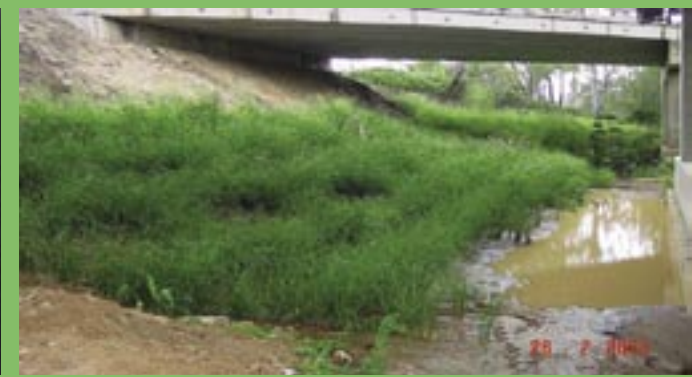
Australia - this river bank and bridge abutment have been stabilized with vetiver. Vetiver is an excellent interface for concrete and soil
