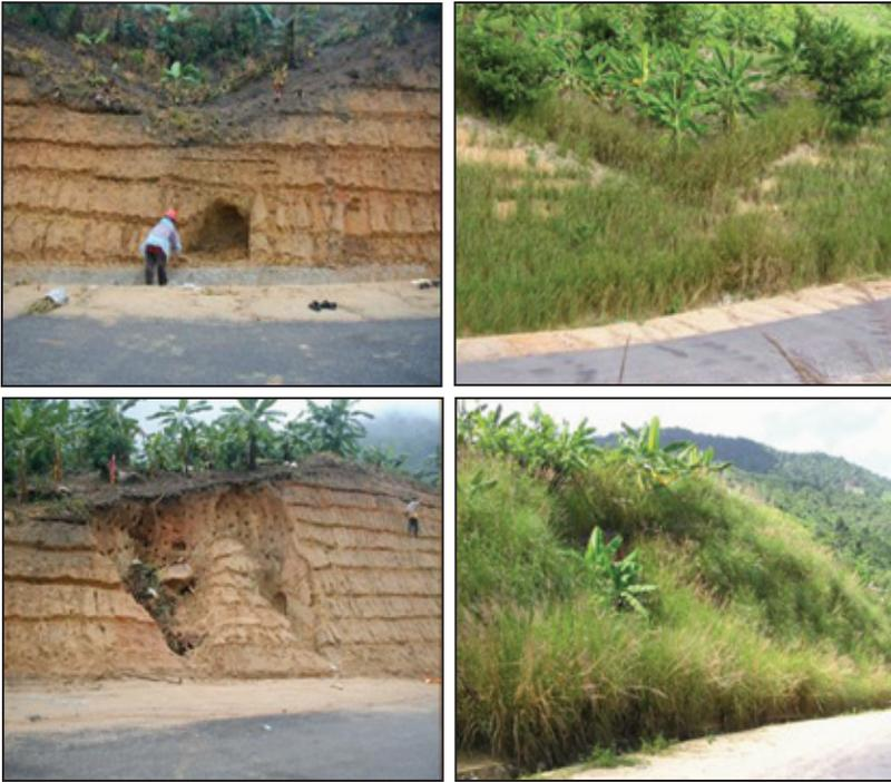
**Photo 28: Pham Hong Duc Phuoc, a road protection project in Khanh Hoa province, road to Hon Ba): left two photos: severe erosion on newly built batter occurs after only a few rains; right two photos: eight months after vetiver planting: Vetiver stabilized this slope, totally stopping and preventing further erosion during the next wet season.**
