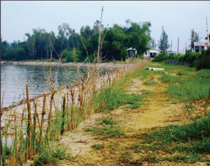
**Photo 9: Upper: March 2002: VS trial at the edge of a shrimp pond, where a canal drains flood water to Vinh Dien River; lower: November 2002: mass planting combined with rock riprap to protect bank along Vinh Dien river.**
