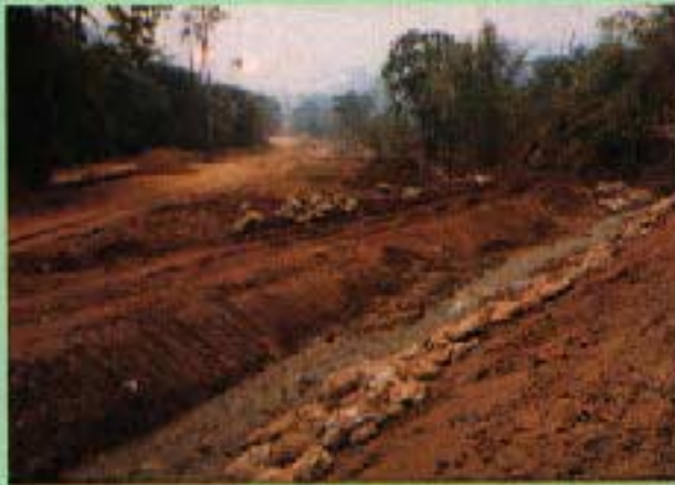
PK 14 + 078: Photo taken in March 1998 (left) and January 1998 (right) After back-filling reinstatement and arranging rocks along the stream
