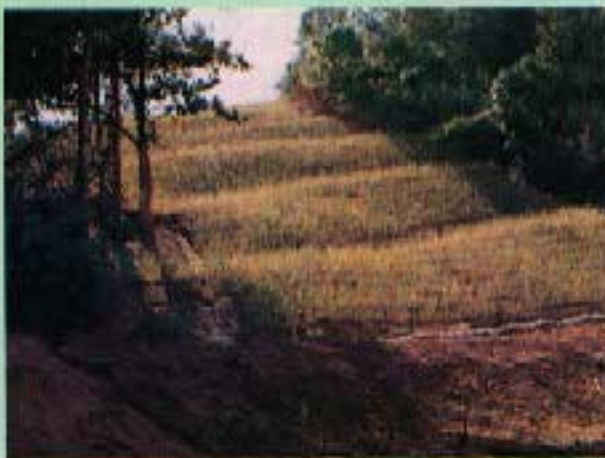
KP 12 + 280: Photo taken on July 1997 (left) and November 1999 (right). On a steep terrain where Ladder berms were built and vetiver grass was planted to prevent erosion.
