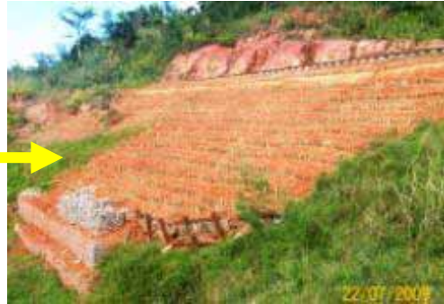
Slopes stabilization under technical criteria of Vetiver System Technology (small drainage included)
