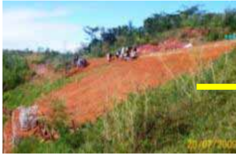
Slopes stabilization under technical criteria of Vetiver System Technology (small drainage included)
