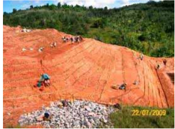
Slopes stabilization under technical criteria of Vetiver System Technology (small drainage included)
