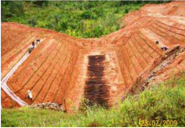
Slopes stabilization under technical criteria of Vetiver System Technology (small drainage included)
