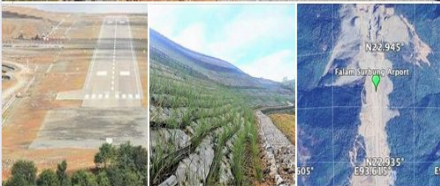
Stabilization of runway 3 m vetiver plants grown by small nurseries
