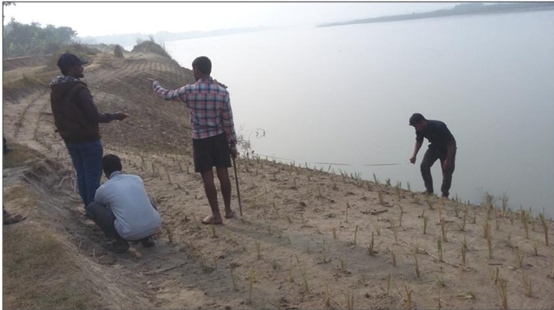
Planting of vetiver in the river bank of the Ganges in different row spacing
