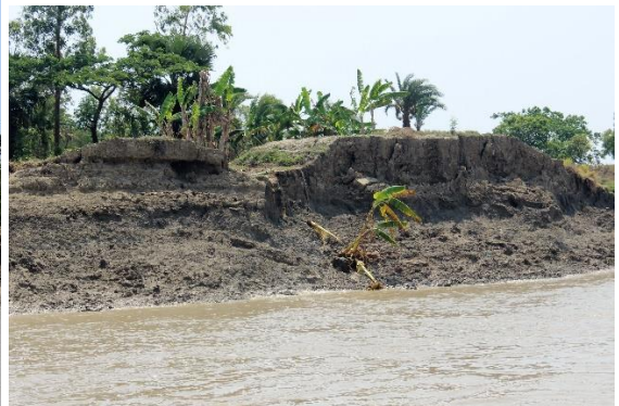
Eroded Protection dike on GHORAMARA Island
