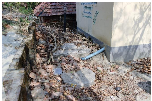
Village Community toilet front and back, discharge effluent to village pond
