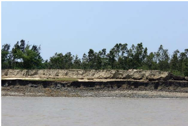
Eroded Protection dike on GHORAMARA Island
