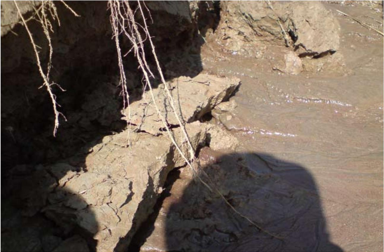
**Telehi, Assam, October 2009, a steep section of the bank that failed, note water seepage at the base of the slope from adjoining ground and length of Vetiver roots recovered from the failed area**
