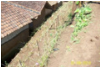
February 2011, Vetiver system in protect community housing, at Buleud, 3 days old.
