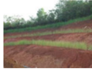
4 months AFTER vetiver plant, Pontianak-Kalimantan Project owner : PT Waskita Karya Project name : Tayan Balai Bekuak Road Population : 50,000 slips Planting start : February 2010
