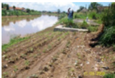
Support ADB project on March 2009 in supply and plating vetiver (65,000 slips) at Citarum riverbank. BEFORE vetiver system implemented
