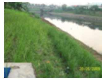
12 weeks AFTER vetiver system implemented
