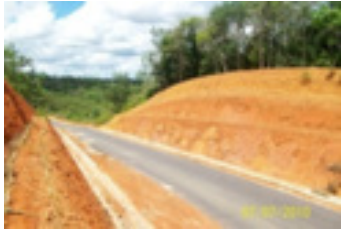
Supply, plant and maintenance vetiver system at Pontianak-Kalimantan for PT WIKA with high Bouksit soil, 5 days old
