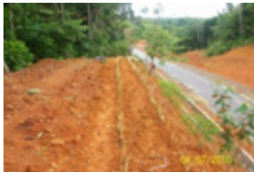
Vetiver system at Pontianak-Kalimantan for PT WIKA with high Bouksit soil, 2 days old
