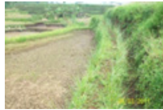
Vetiver system application on small ditch at BULEUD area, Garut, 2 months old
