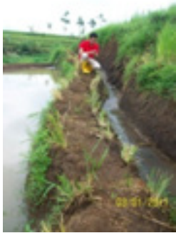
Vetiver system application on small ditch at BULEUD area, Garut, 5 days old
