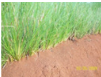
A year AFTER vetiver system implemented at Lingkar Nagreg road sloping
